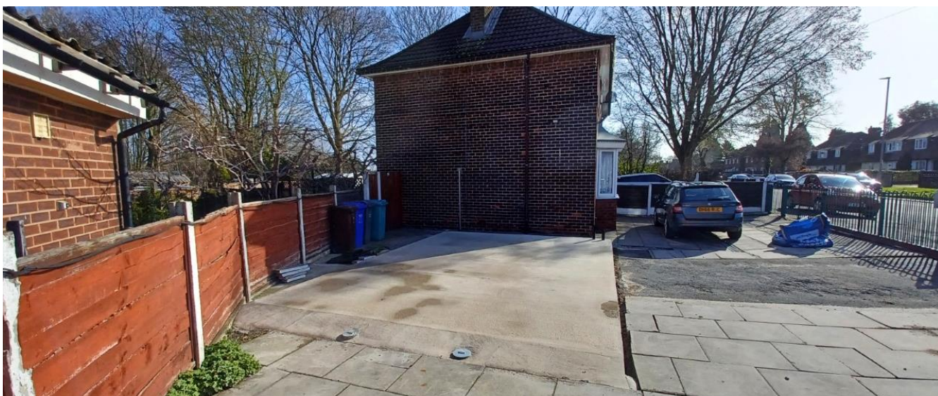
Figure 3. View of the foundations of the proposed development.
