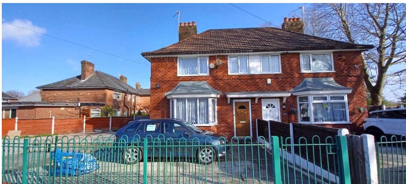
Figure 1. Principal elevation of No.257 Hollyhedge Road.
