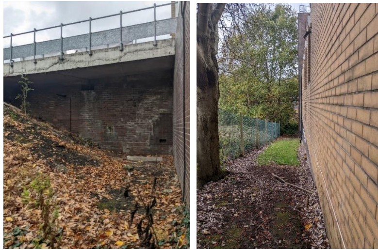
Figure 4: Photographs showing the steep western slope along the western site boundary with the basement wall, looking north, with a pedestrian bridge across the slope (left) and a gentle slope along the southern site boundary, looking west (right).
