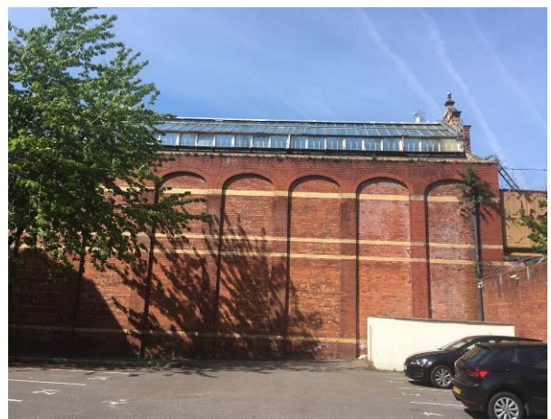
The east elevation of the Females pool, note restrained detailing.
