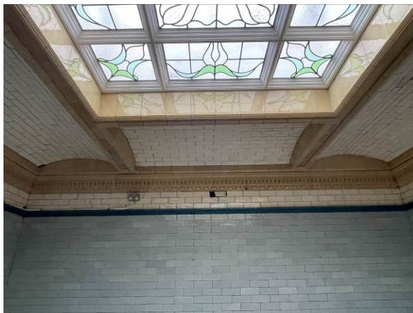
Damaged tiling and previous fixing holes / voids to be utilised for securing detectors in the Turkish Baths
