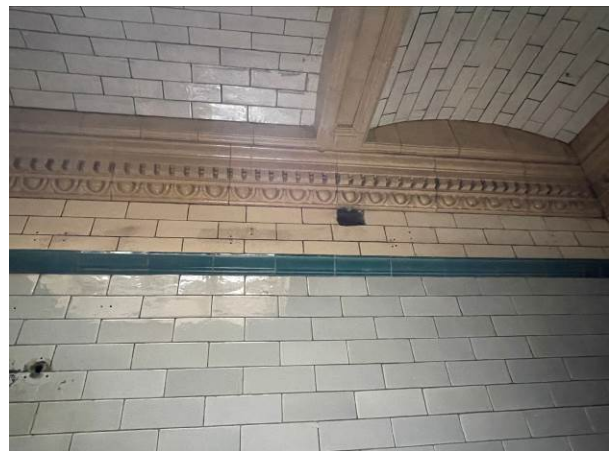
Damaged tiling and previous fixing holes / voids to be utilised for securing detectors in the Turkish Baths
