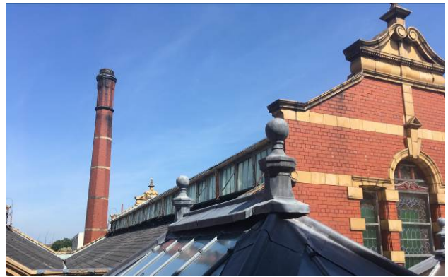
Pool Hall roofs with slating beneath full length lanterns and gables with Venetian windows.
