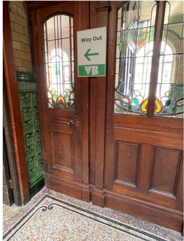
Manual call points to be fitted to architraves at final exits (L) and in recesses in screens outside lobbies (R)
