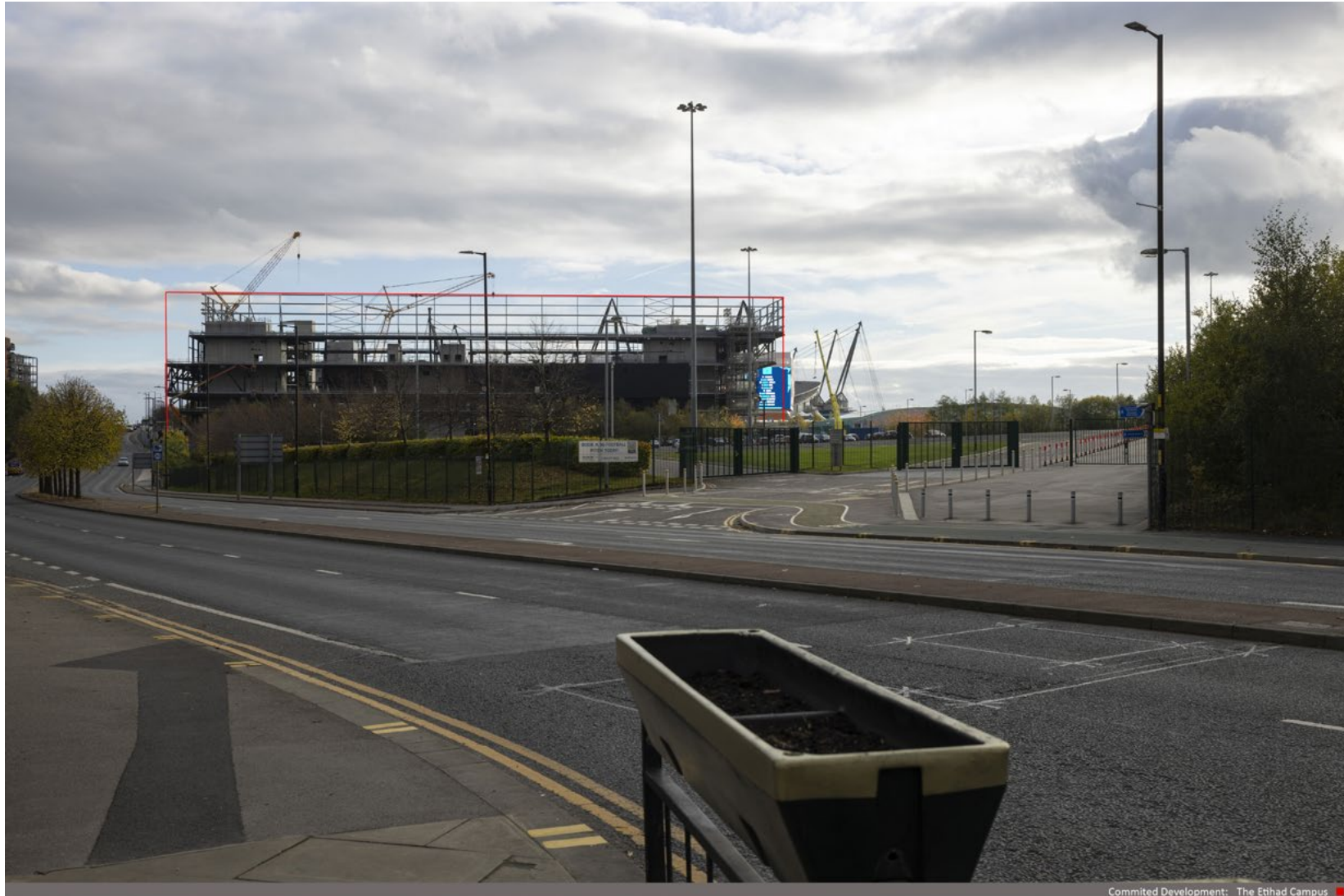
View 9: Photomontage | View south towards site from pedestrian crossing on Alan Turing Way A6010, at junction with Brisco Lane.
