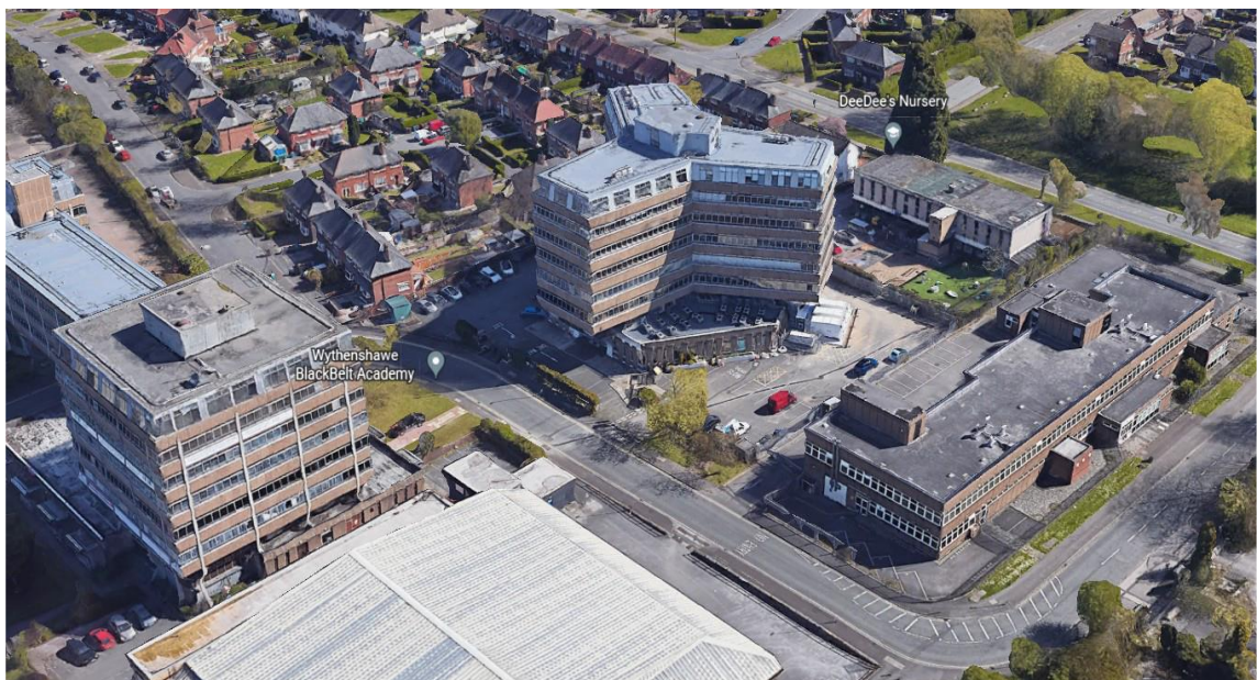
Figure 2: Existing building and surrounding context
