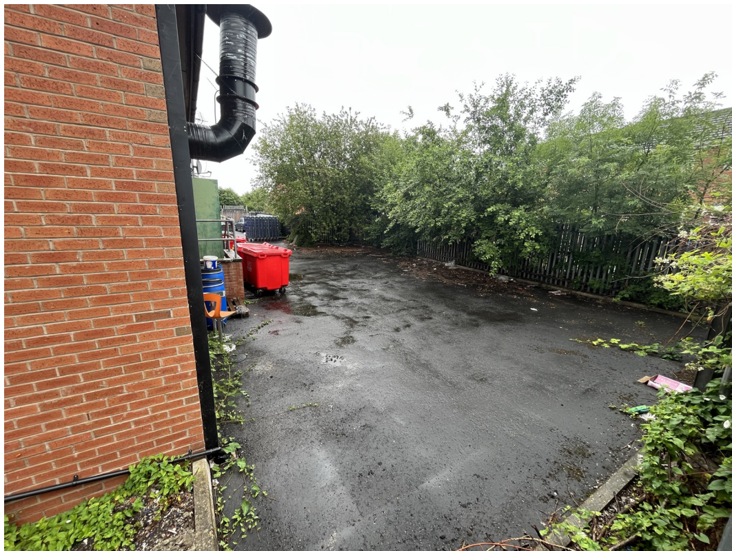
Figure 3. Rear service yard
