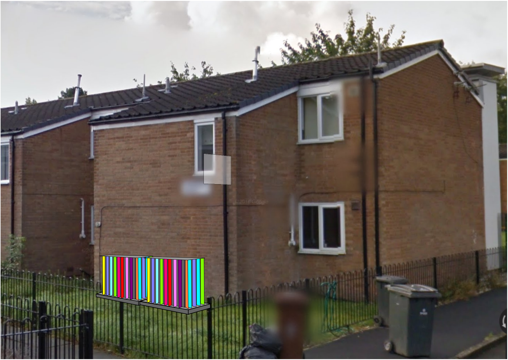
Proposed typical arrangement for heat pump ventilated enclosure, partially obstruction the heat pump.
