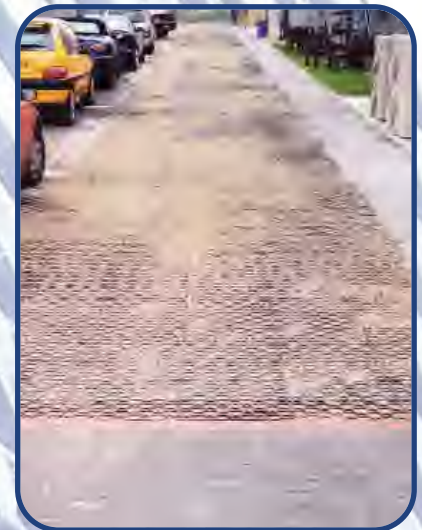
Car Park Infiltration Area.
