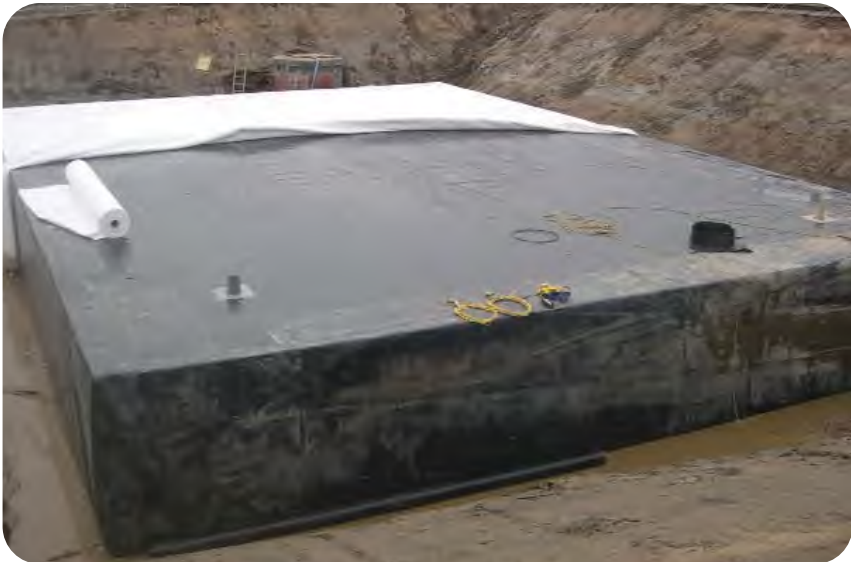
2mts deep tank with 3mts cover
