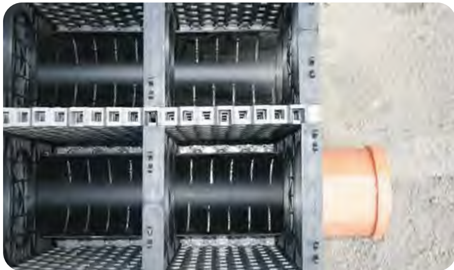
Top view showing low flow maintenance channel.
