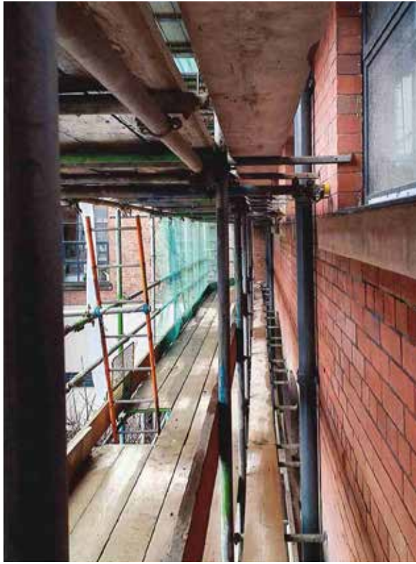
Image of system in use on listed building, (above) the narrow walkway close to the building, and (below) self tapping anchor eye-bolt fixed through mortar as a reversible fixing
