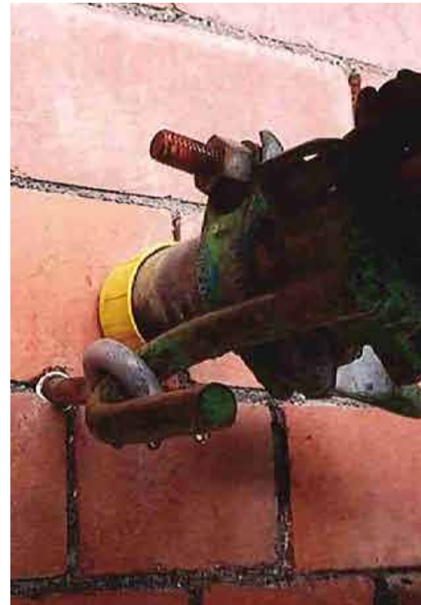
(above) right hand side the horizontal scaffold pole abuts the building and is hooked on (below) into the bolt to minimise contact with the fabric
