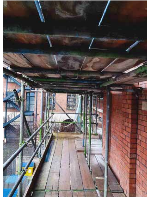
(above) right hand side the horizontal scaffold pole abuts the building and is hooked on (below) into the bolt to minimise contact with the fabric
