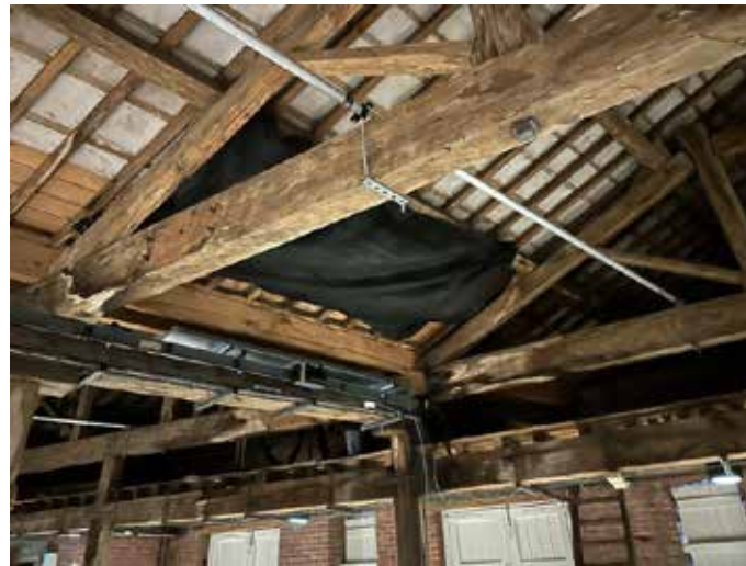
Evidence of existing services along internal roof structure
