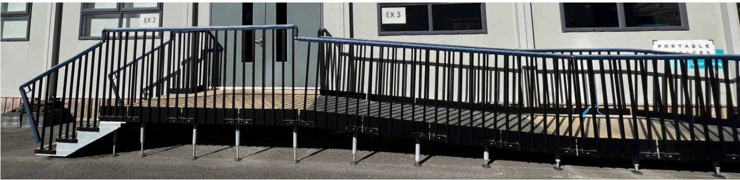
Unit C - Access Ramp
