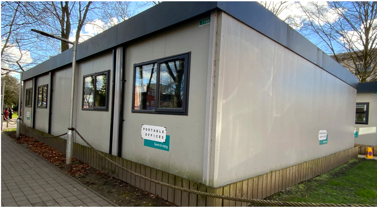
2. Unit C - Double Storey, Double Classroom
