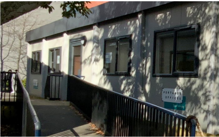
Unit A - Windows and Doors (West Elevation)
