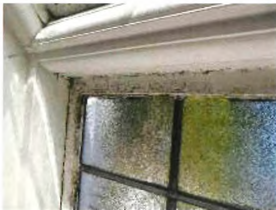
Single glazed window and timber window frame
