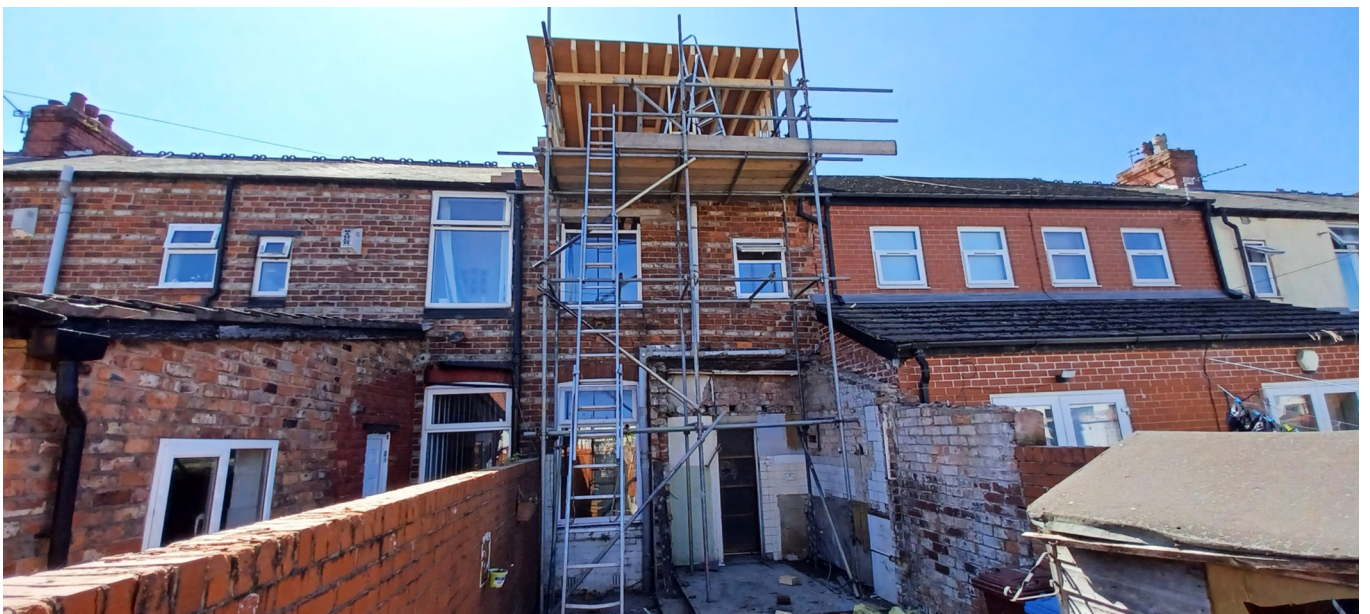
Figure 3. Rear roof of property.
