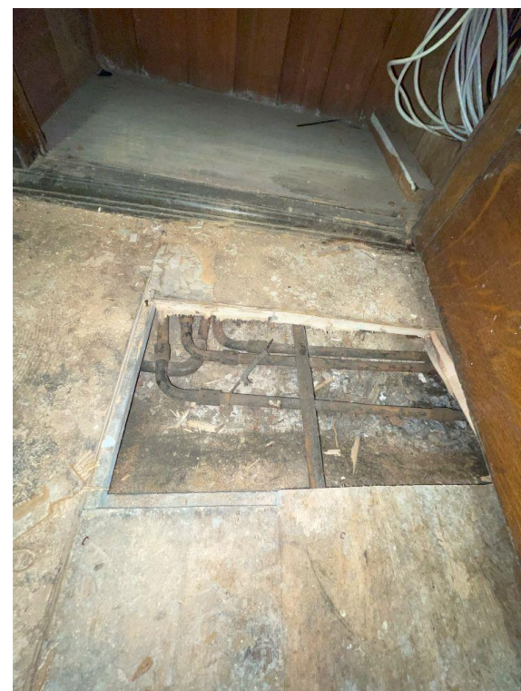
Detail of floor
