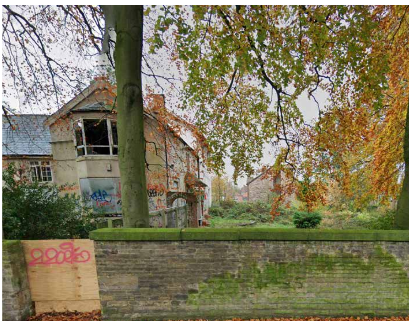
OVERGROWN LAND TO NORTH OF BUILDING
