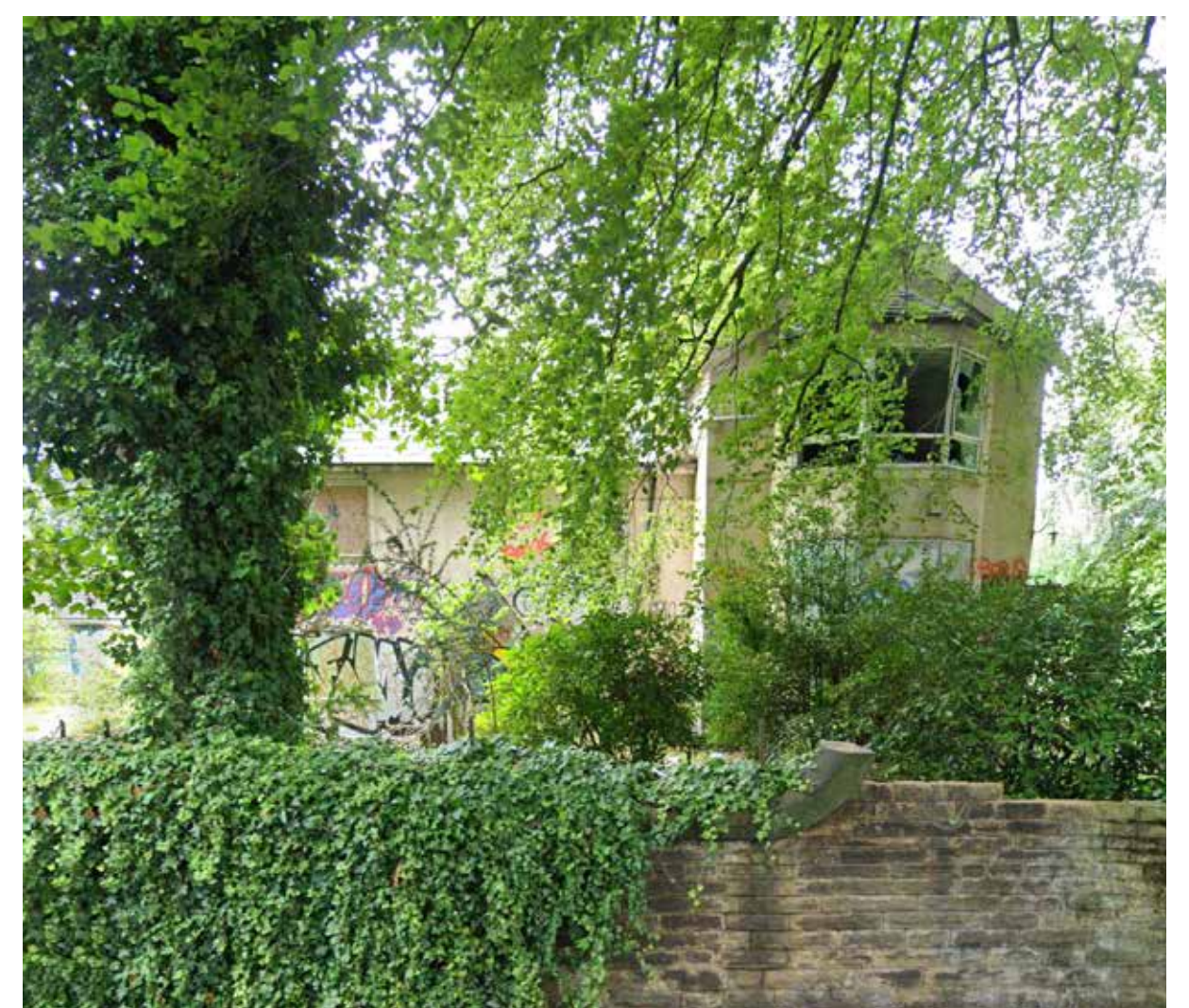
WALTON COTTAGE VIEW FROM WITHINGTON ROAD
