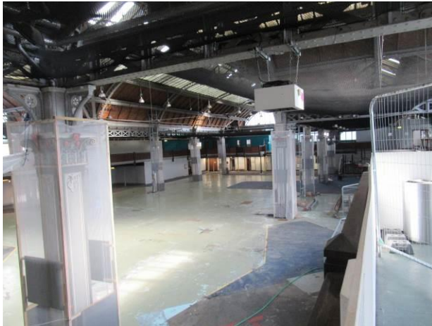
General view internally
