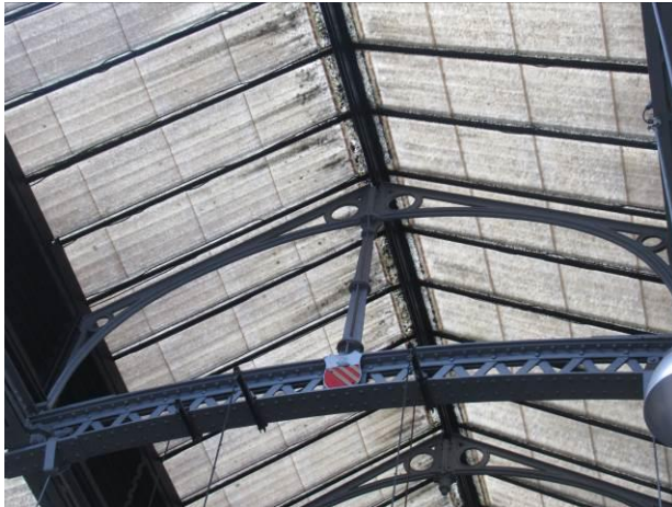
View on apex detail for centre aisle trusses, showing vertical member
