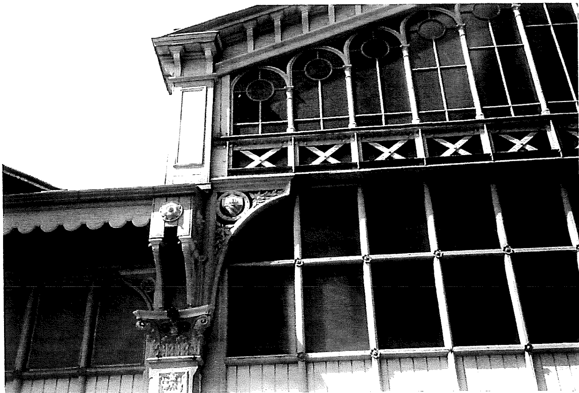
View of an ornate cast iron bracket supporting the Eastern Gable WI Lattice Girder.
