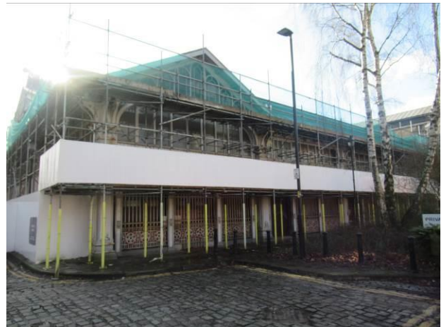
General view on rear elevation from Byrom Street
