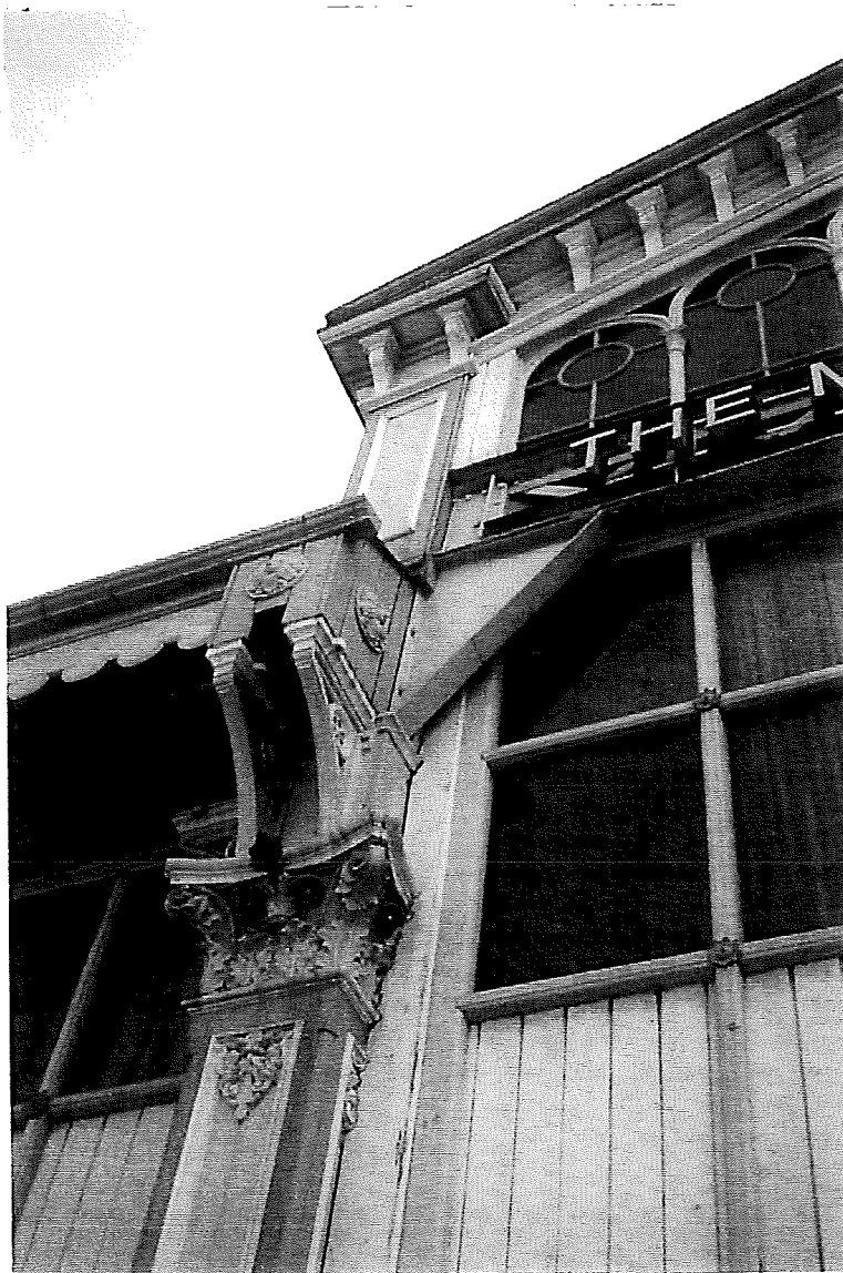
View of an ornate cast iron bracket supporting the Eastern Gable WI Lattice Girder.
