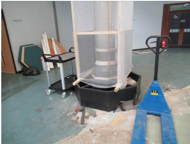
Local box out and tanking to the base of columns where water ingress has been historically observed
