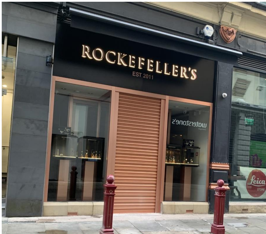
Works to the shop front as part of this application
