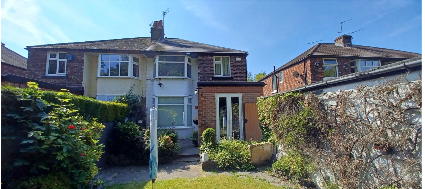
Figure 2. Rear view of property.
