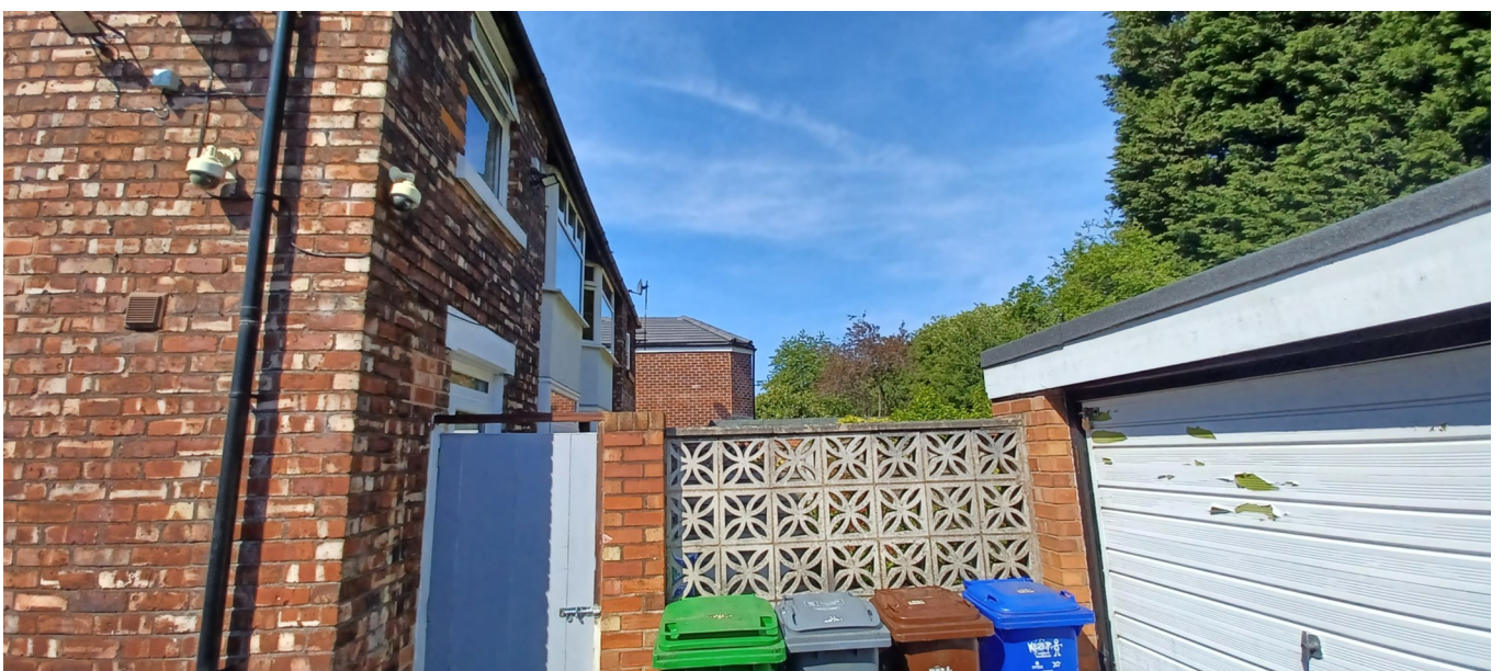
Figure 7. View of similar extension along Mauldeth Road West.
