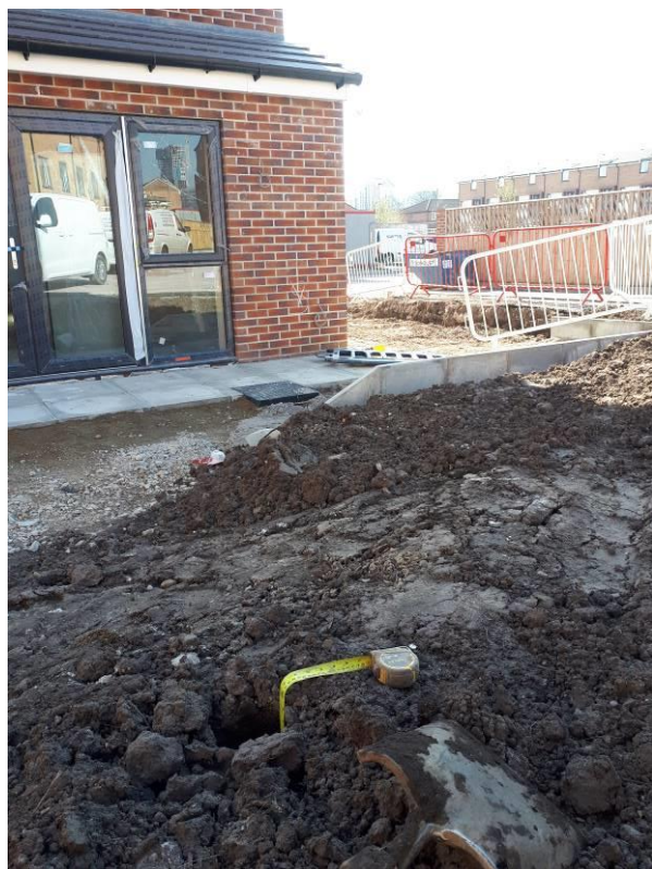
Photograph 7: Plot 289 Validation Pit 2 Location
