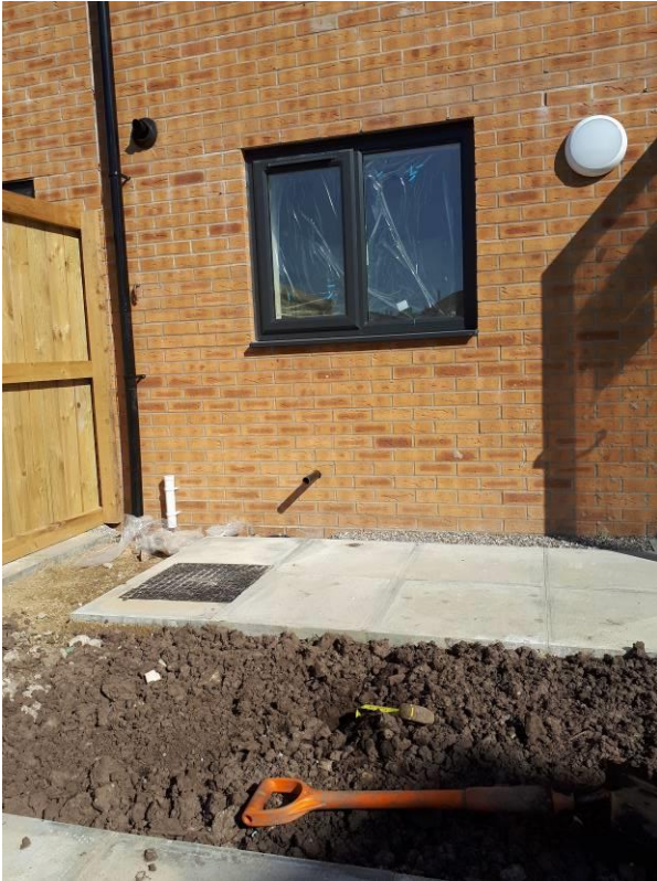
Photograph 1: Plot 284 Validation Pit 1 Location
