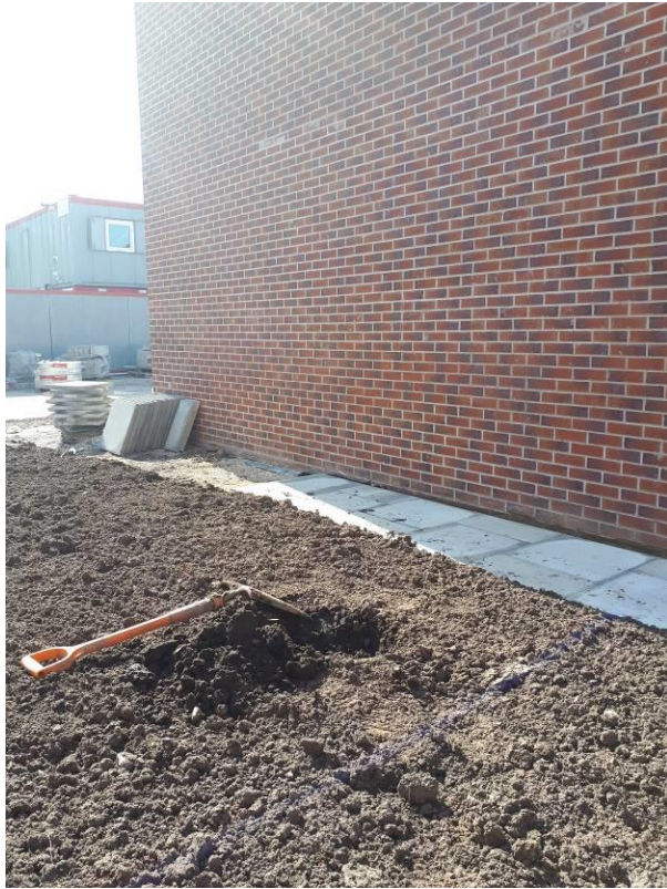
Photograph 5: Plot 289 Validation Pit 1 Location
