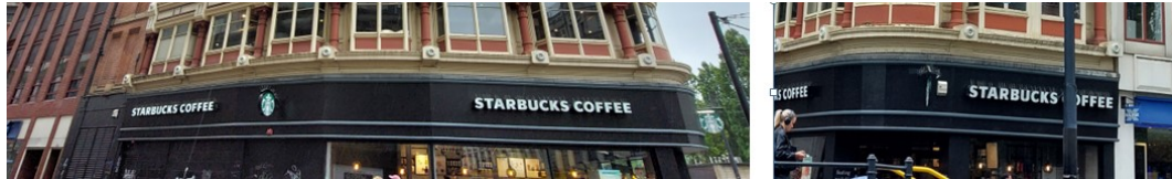
Plate 17: The existing wordmarks to the fascia.
