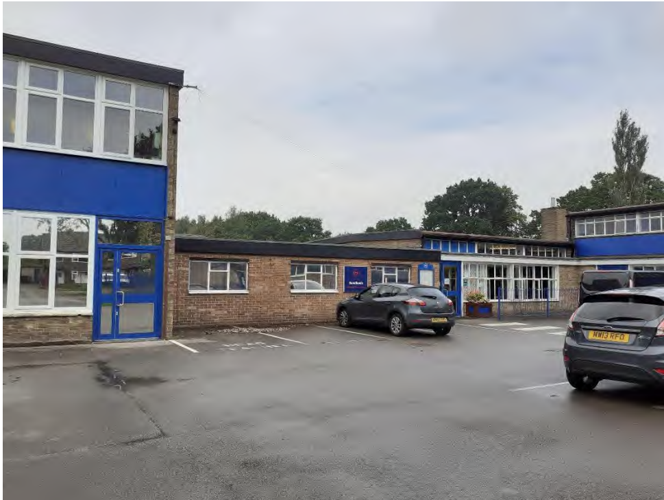
Photograph 1- Showing the front of the existing school buildings.
