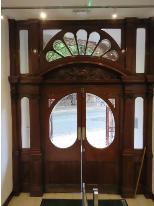
Figure 37: The original Art Nouveau hardwood entrance doors and glazed screen onto Chepstow Street.
