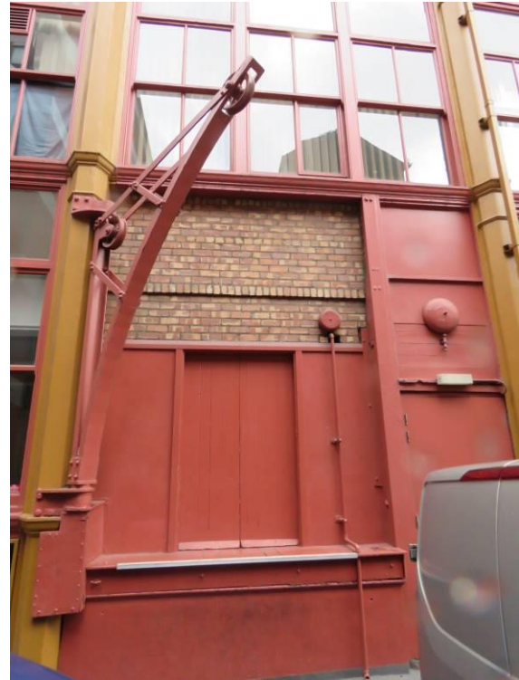
Figure 35: One of the two original teagles (hoist) and loading bays on the side street to the east.
