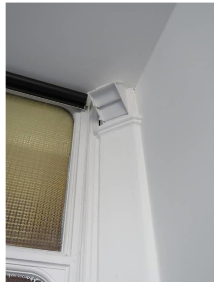
Figure 52: An example of one of the octagonal cast iron columns showing the integral ventilation system as seen when the column is used for partition walls, allowing for individual vent outlets to vent different rooms.
