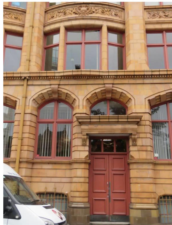
Figure 33: The former entrance on Chepstow Street South which was originally designed to be used by other tenants occupying the building.
