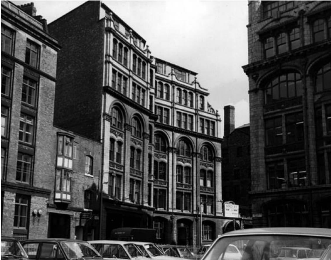
Figure 5: Looking east along Chepstow Street in 1973 before the street was re-routed across the surface car park in the mid-1980s. Canada House can be seen to the extreme right whilst H. S. Booth's Block C, also designed by W & G Higginbottom in 1904 can be seen to the centre. Note the striking similarity between the two buildings. (Source: Manchester Archives)
