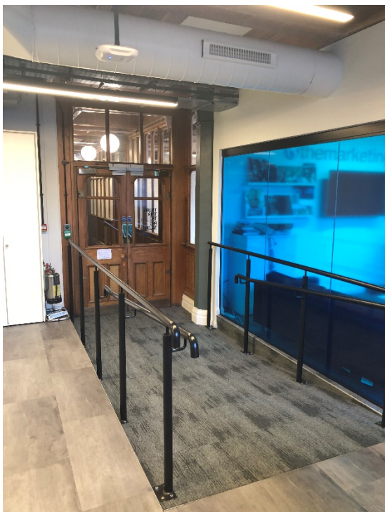
Fig. 5. And 6. Views of the entrance (left) to the office unit with original door and glazed partition and modern ramp, handrail, partitions, raised access floor and floor finishes.
