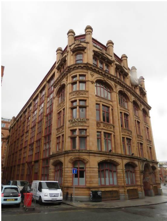
Figure 29: Looking south-east towards the entrance front of the building, showing the district change in style and decoration between the principal front (right) and service side of the building (left).
