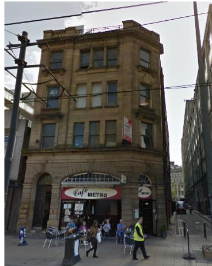
Figure 23: 20-22 High Street – 1915-17 W & G Higginbottom, Unlisted
