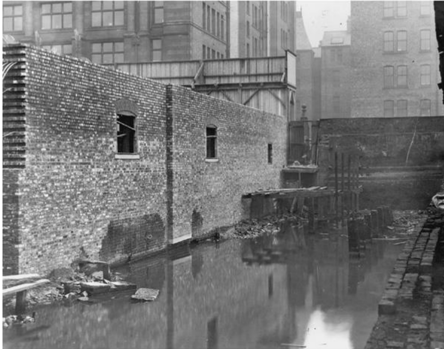
Figure 14: A view looking south-east along the former branch canal arm showing the construction of the foundations and basement level of the new Hippodrome Theatre on Oxford Street being constructed in 1904 following the demolition of F. W. Sephton's glass works. The building in the left background is the side of Tootal, Broadhurst & Lee's warehouse. Note the abrupt termination of the branch canal arm as it reaches the line of Great Bridgewater Street to the right. The east elevation of Canada House would be late built on the line of bricks to the right of the image and the branch arm would become the private side street to the east of the building. (Source: Manchester Archives)
