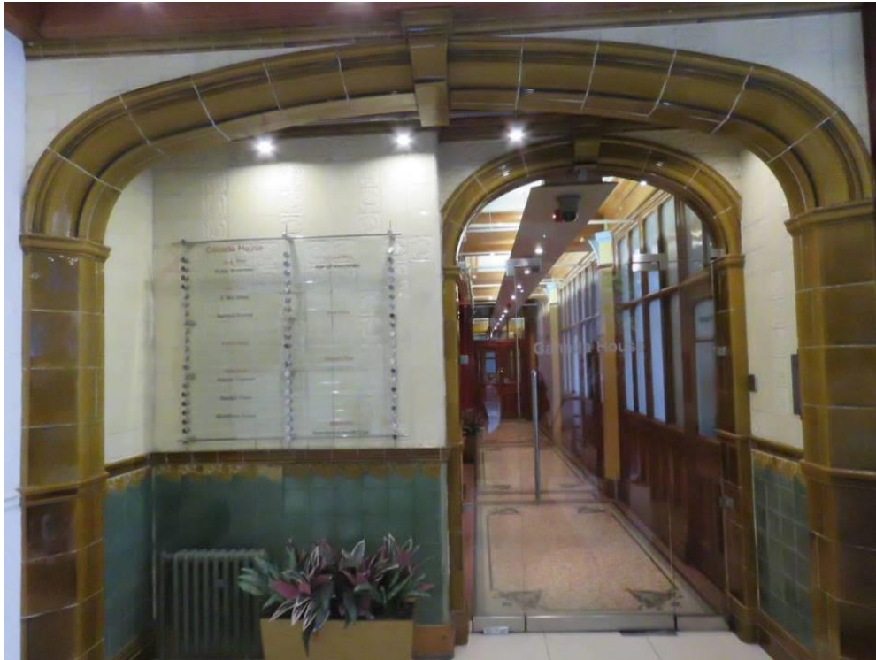
Figure 36: The original glazed terracotta archway and glazed tiles of the entrance hall, looking through into the main ground floor corridor.
