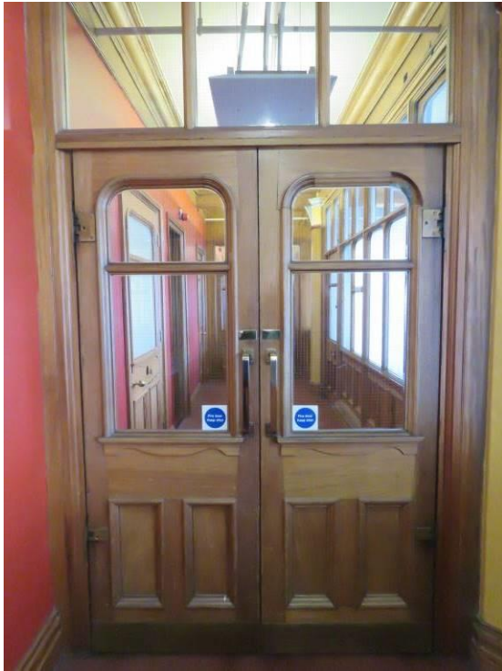
Figure 55: An example of the original glazed swing doors found on each main corridor.
