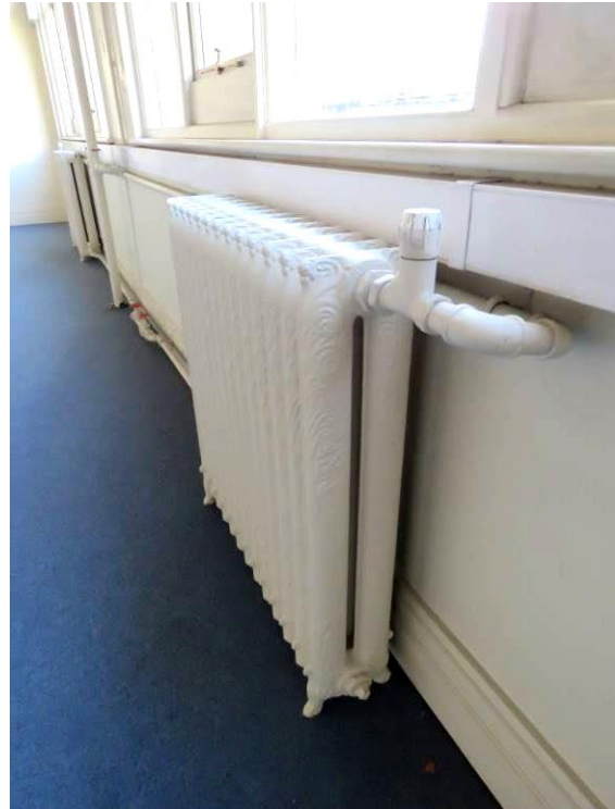
Figure 56: An example of the original decorative cast iron radiators.
