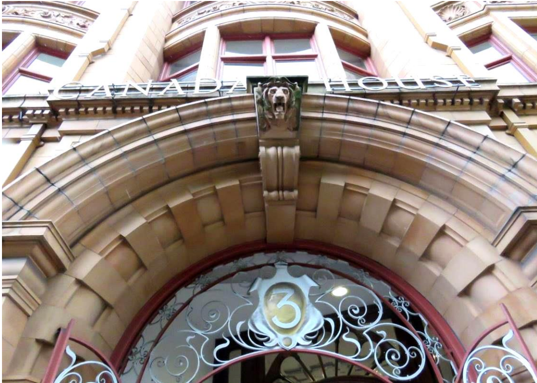
Figure 31: The elaborately ornate Art Nouveau wrought iron entrance gates and early-20 th century 'Canada House' sign.
