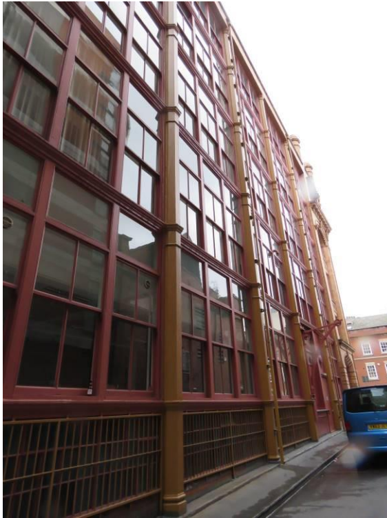
Figure 34: Looking north along the rear side street showing the entirely glazed eastern elevation which originally formed the warerooms on each floor.
