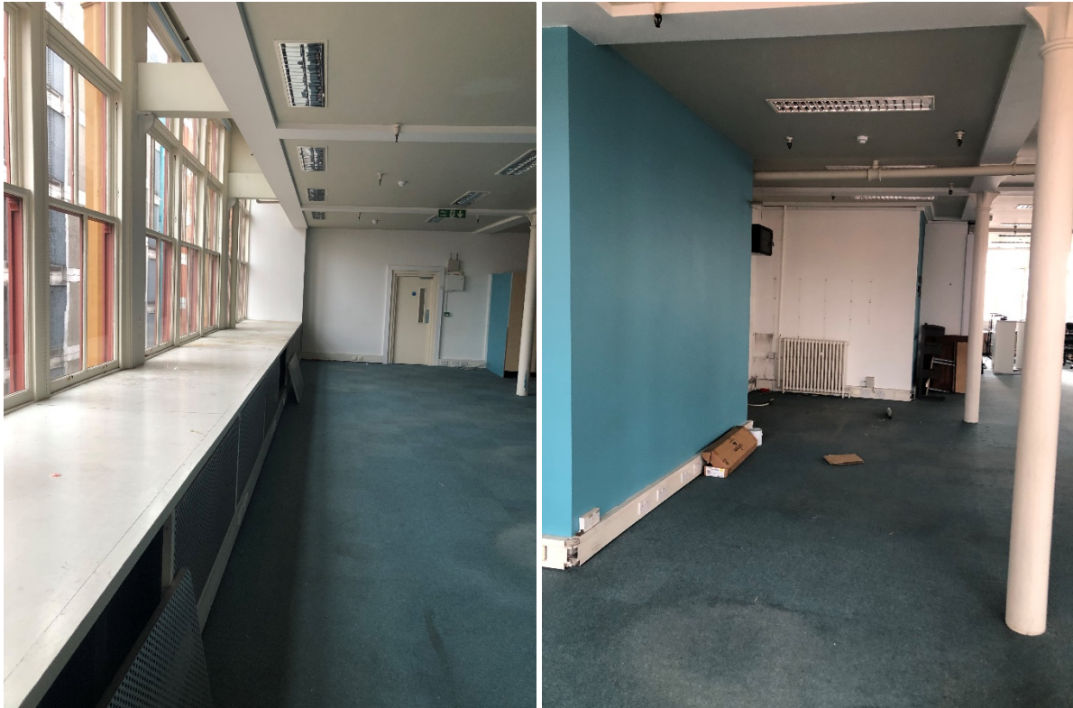
Fig. 1 and 2. General views through the 3 rd floor office unit. The boxing in adjacent to the window covers the original cutting tables. Note the modern dropped ceilings and exposed original cast iron columns.
