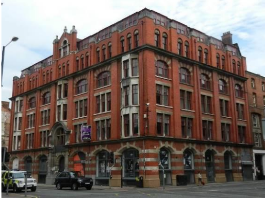
Figure 18: 29-31 Dale Street - 1908 W & G Higginbottom, Grade II
