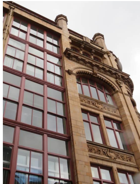
Figure 30: A detail of the district and clear change in style and materials between the principal and functional parts of the building as seen from the rear side street (east). The full-height windows to the left are fitted between the exposed iron frame of the building and allowed much more light to enter each wareroom.
