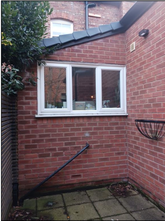
Figure 3: View within rear yard area looking south.
