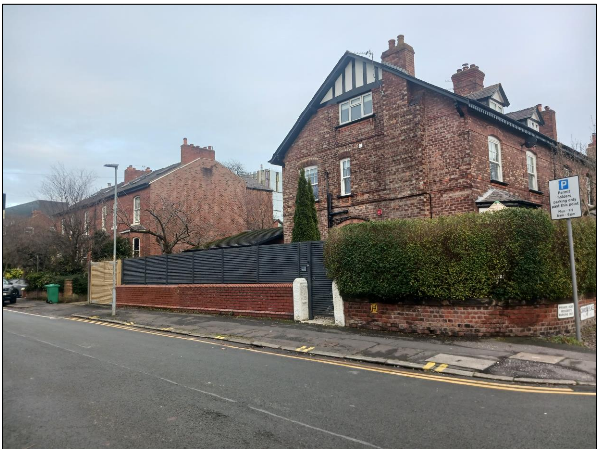
Figure 1: View of 11 Circular Road.
