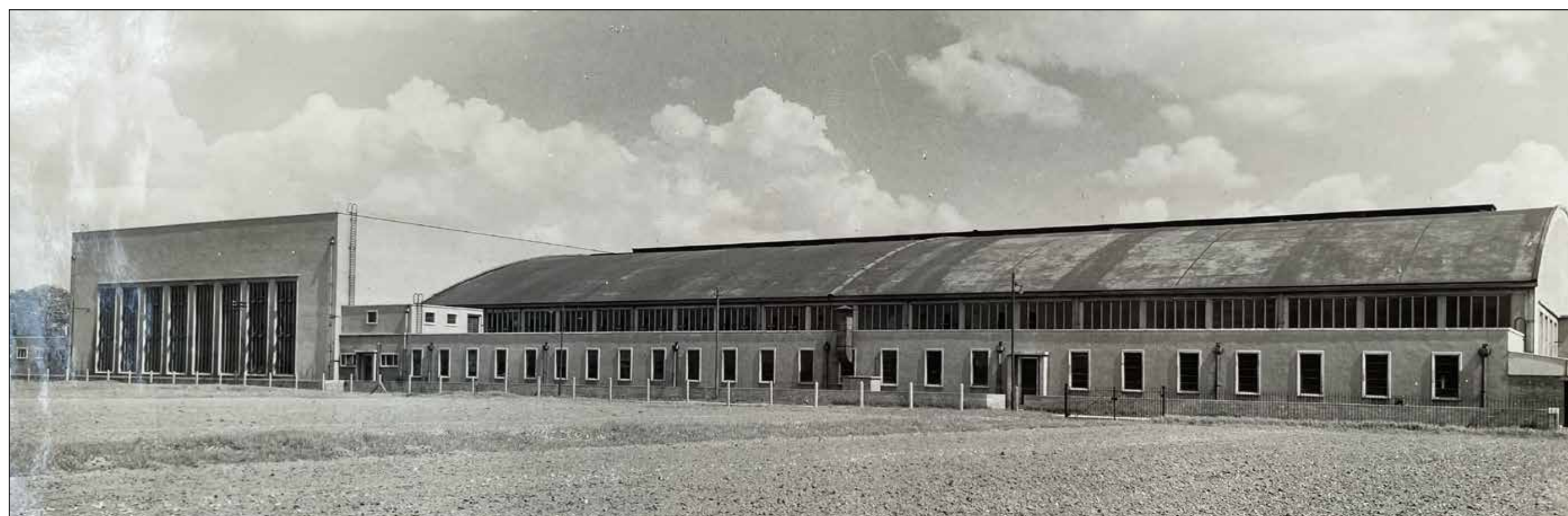
Image 12: Archive photograph from 1950s, showing long side view of exterior, with wings (now demolished).
