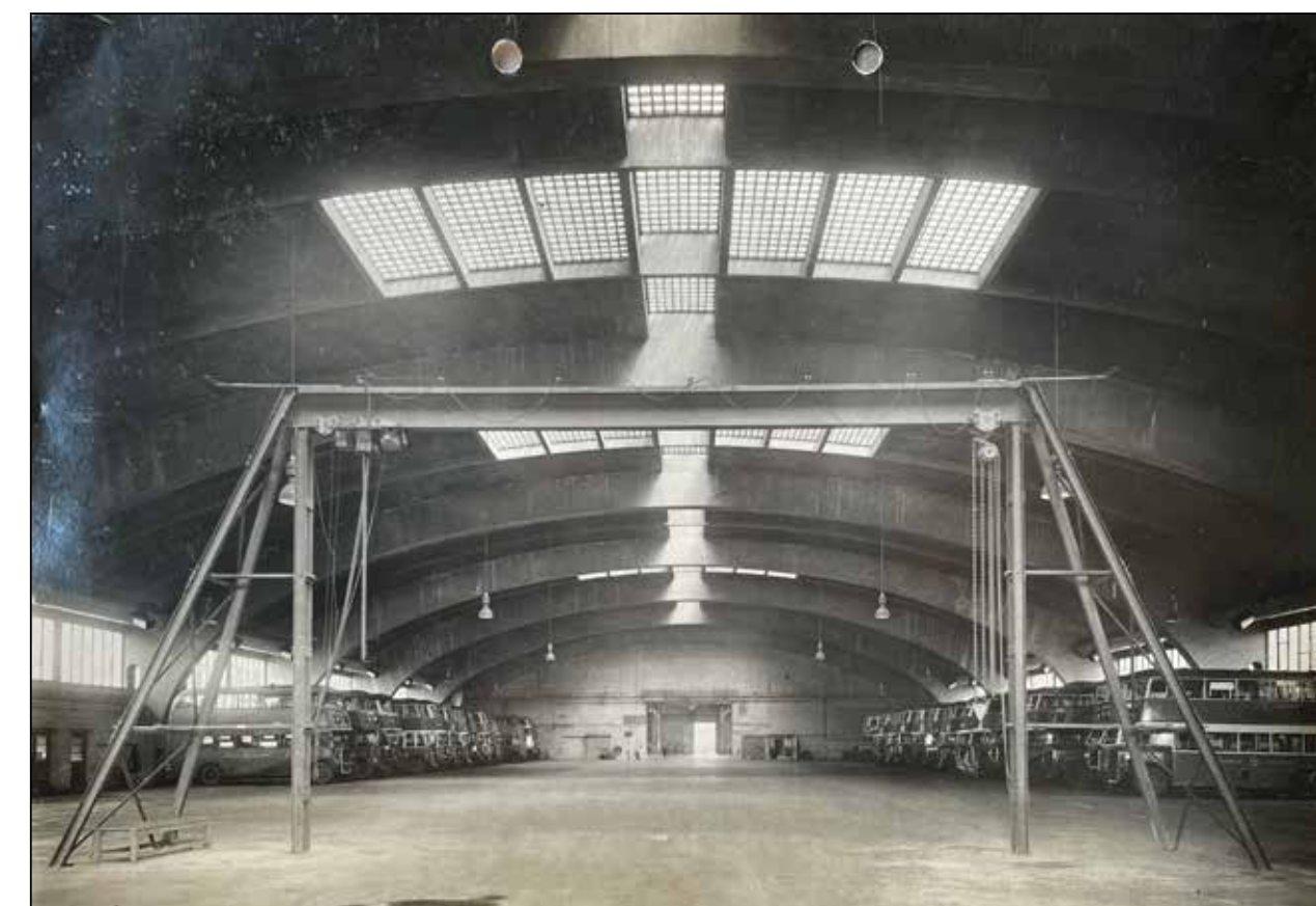
Image 8: Archive photograph showing original rooflights. 1950s.
