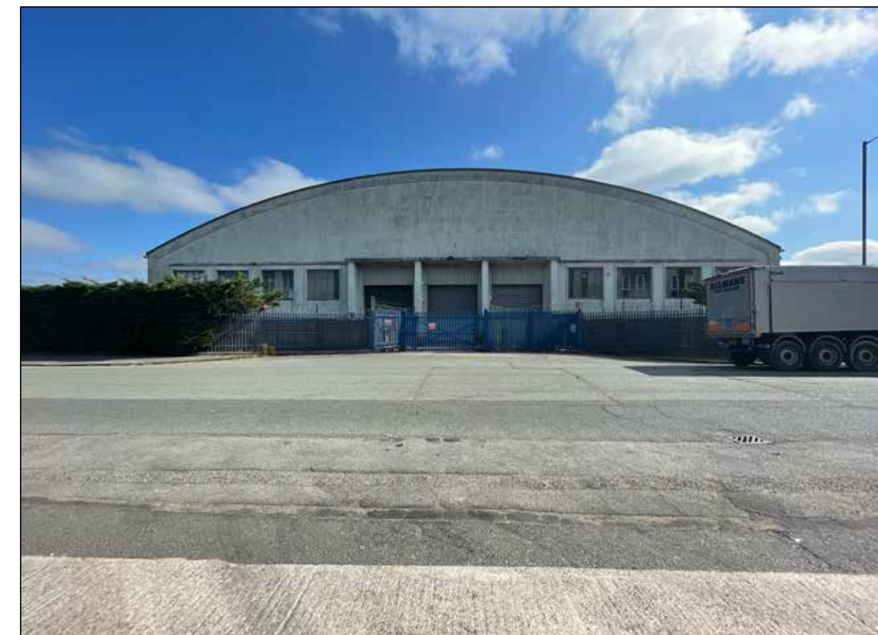
Image 28: External view of garage from Bradnor Road.
