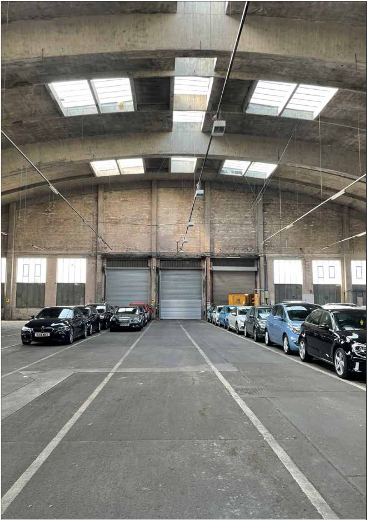
Image 14: Contemporary photograph showing internal roller shutters to front, windows with covering and original brick and concrete structure.
