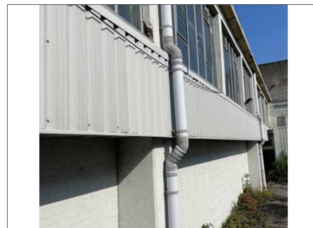
Image 26: External view of over-cladding and modern drainpipes.
