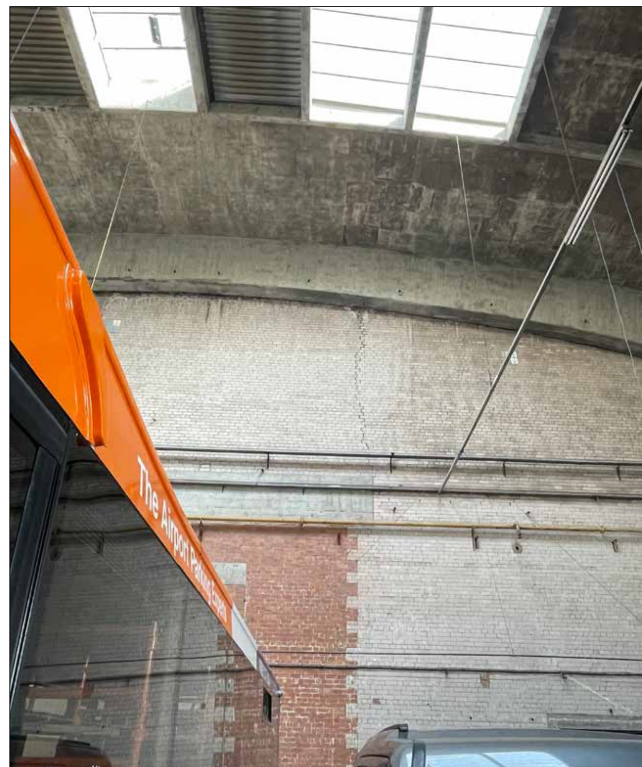
Image 16: Contemporary photograph showing blocking up between front and rear areas of the bus garage.
