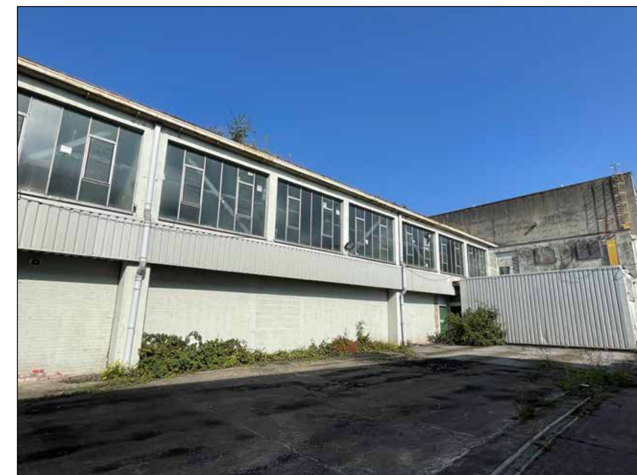
Image 17: Contemporary photograph showing over-cladding of junctions of former wings.
