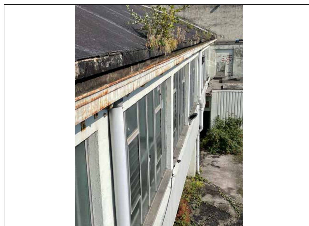
Image 25: High level view of roof covering, gutters and windows to side elevation.
