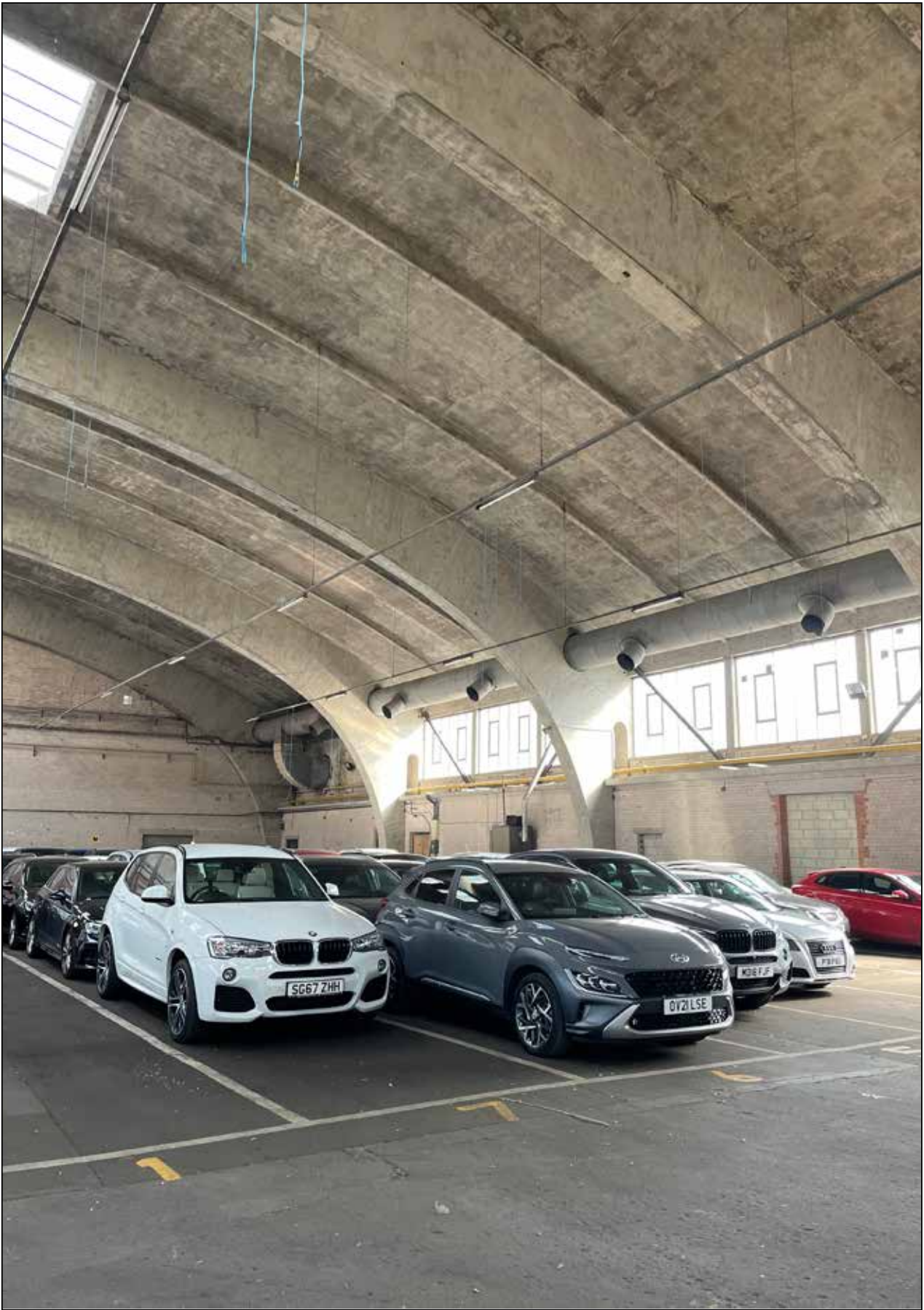
Image 15: Contemporary photograph showing roof and infill to side walls.
