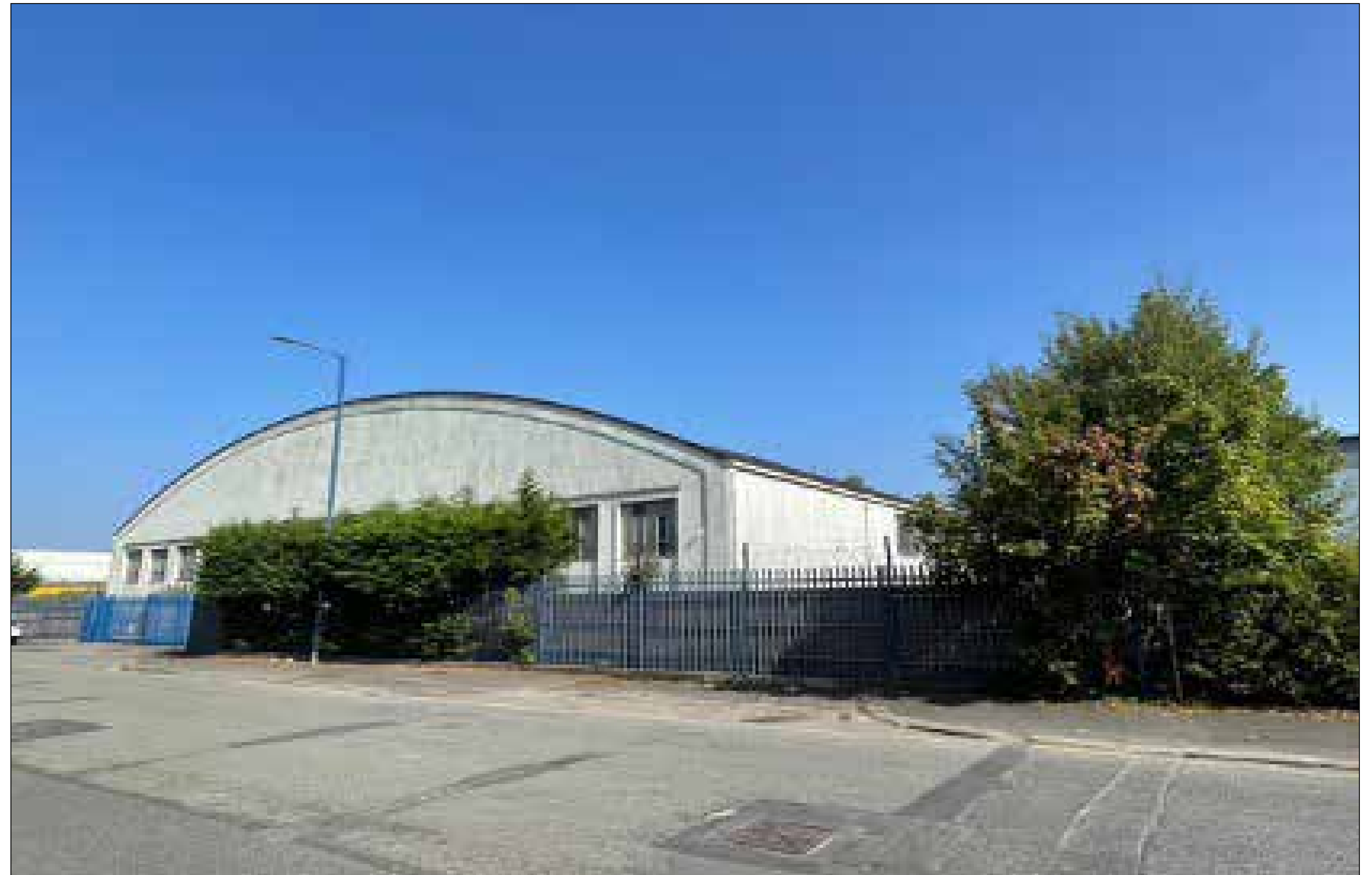
Image 33: View of bus garage from Bradnor Road.
