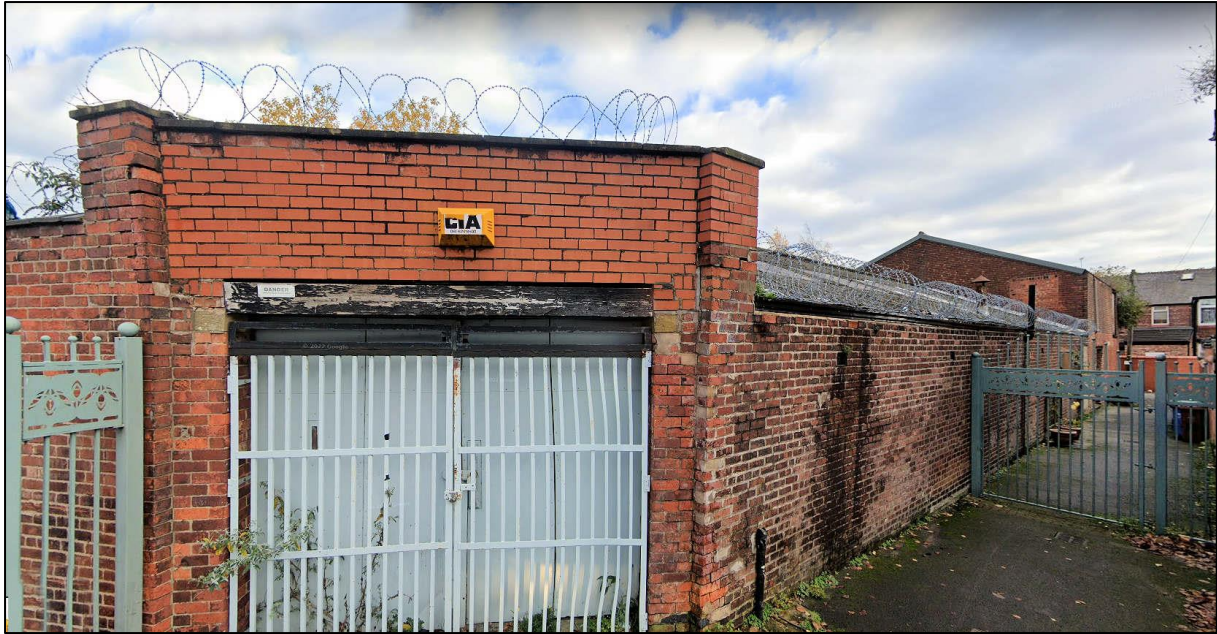
Plate 5: General View of the buildings from Dalton Avenue.
