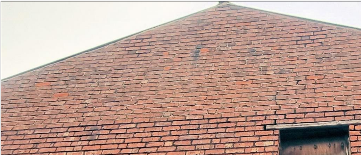
Plate 9: The verges of the southern facing gable were well mortared with no PRFs. Areas of darker missing mortar around the lintels did not provide crevices sufficiently deep for roosting.
