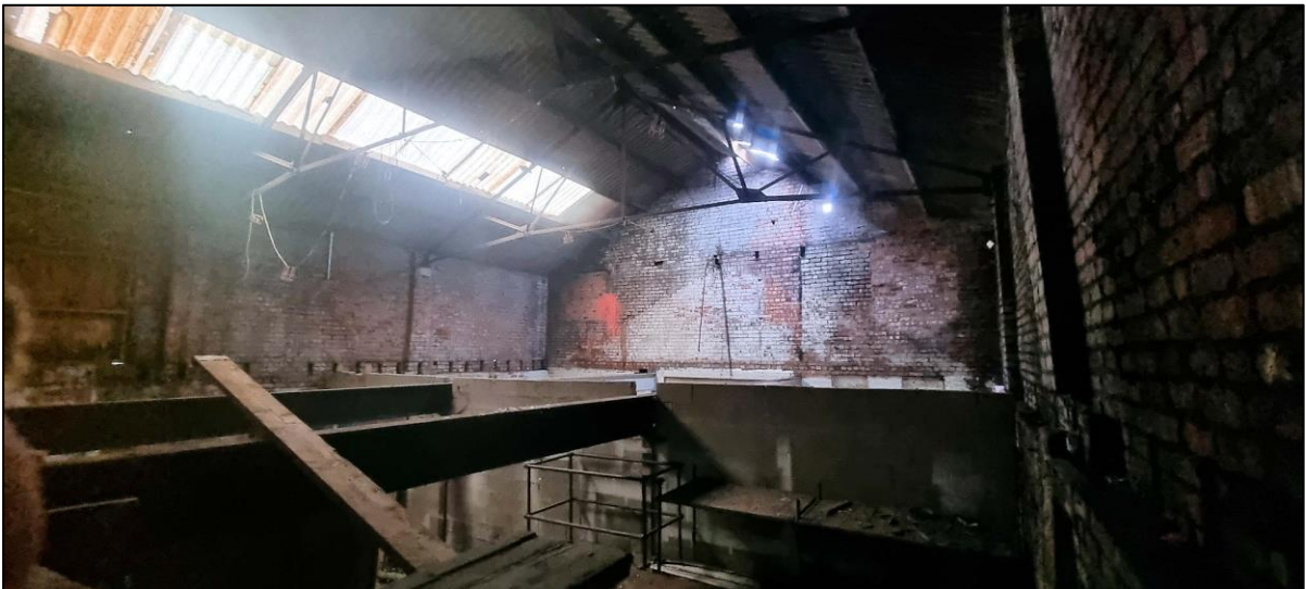
Plate 18: The two-storey building was also a void open from the floor to the roofing sheets and trusses. This offered no roosting potential.
