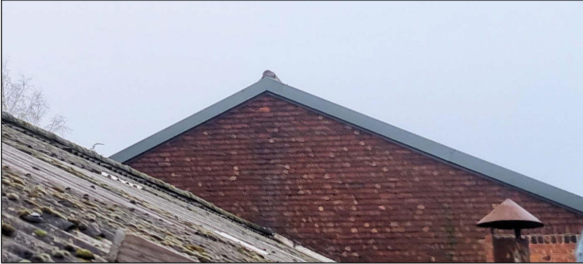
Plate 8: The dry verge boards of the two storey building were afforded close attention as these can harbour roosting bats, but the survey found no gaps and no roosting potential.
