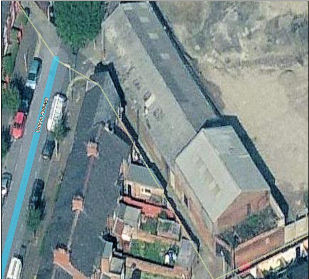
Plate 6: The two roof areas of the former light-industrial building were inspected.
