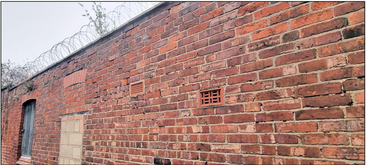
Plate 11: The coping stones on the wall tops were intact with no roosting potential.
