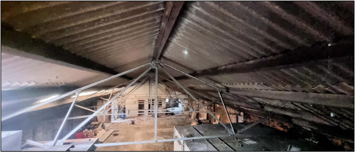
Plate 17: Internal view of the single storey building with exposed roofing sheets and trusses.
