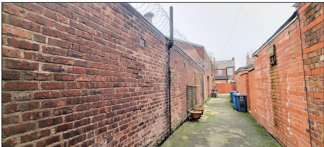
Plate 4: The building and the hardstanding had little floristic value.
