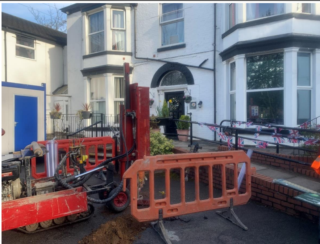
View of the windowless sampling rig at the front entrance, facing northwest
