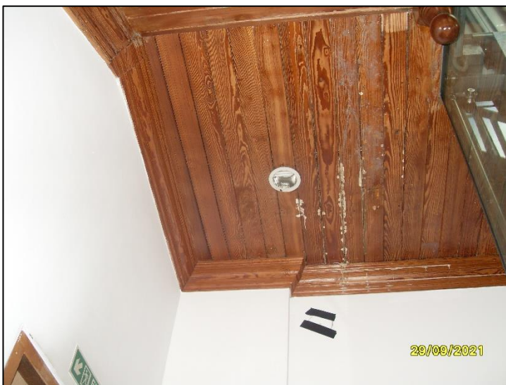
PHOTO 06 – Internal, underside of timber landing (staircase)
