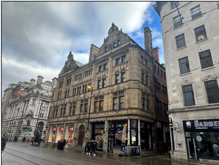
PHOTO 02 – External, junction of Cross Street to Town Hall Lane
