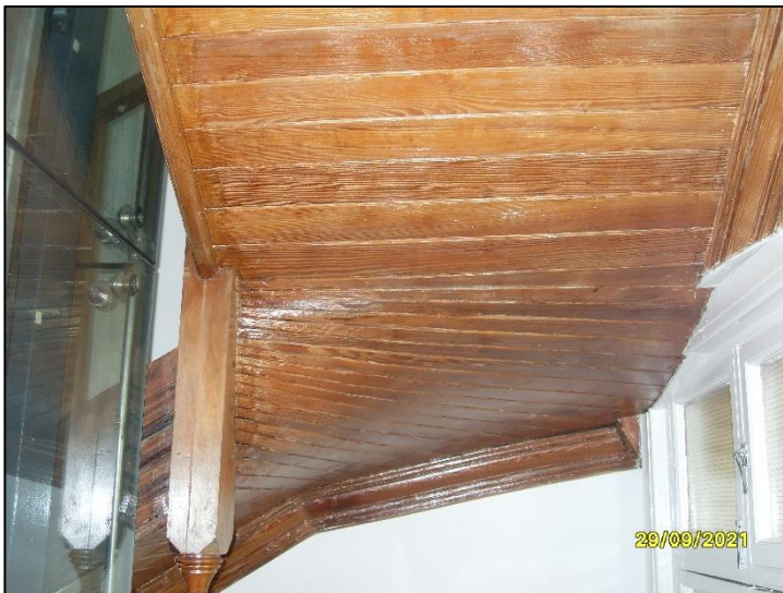
PHOTO 05 – Internal, underside of timber staircase
