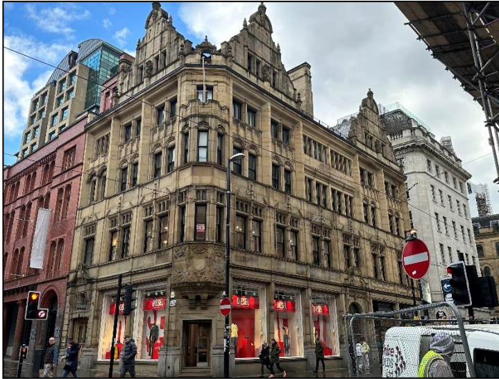
PHOTO 01 – External, junction of Cross Street to King Street
