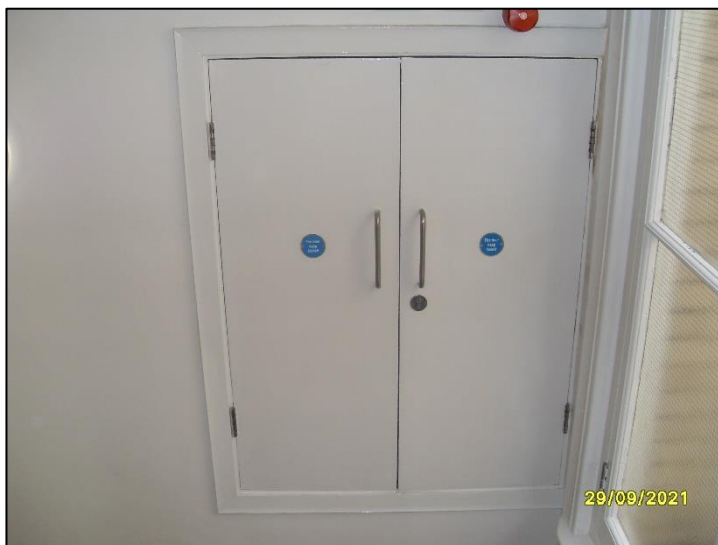
PHOTO 09 – Internal, riser cupboard on communal landings
