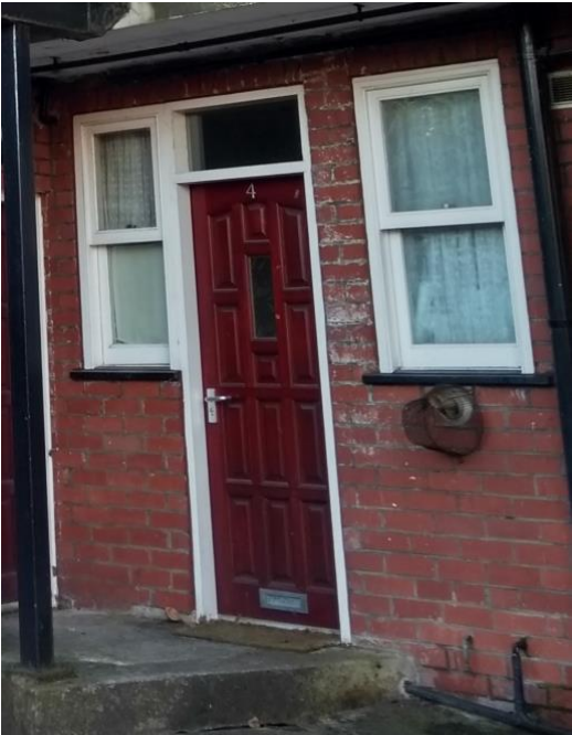
Figure 6. Example of Existing Doors and Windows
