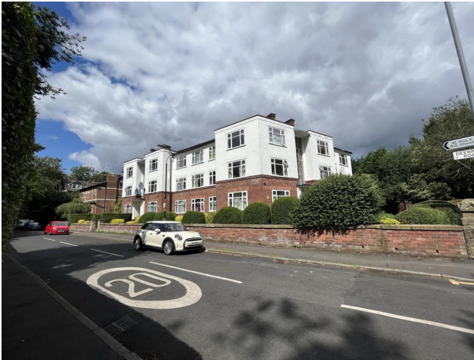
Figure 1. Front (note these windows have been replaced)
