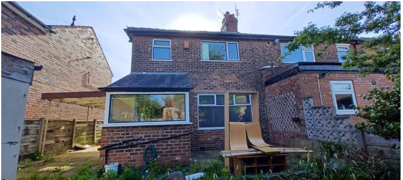
Figure 5. Rear view of property.
