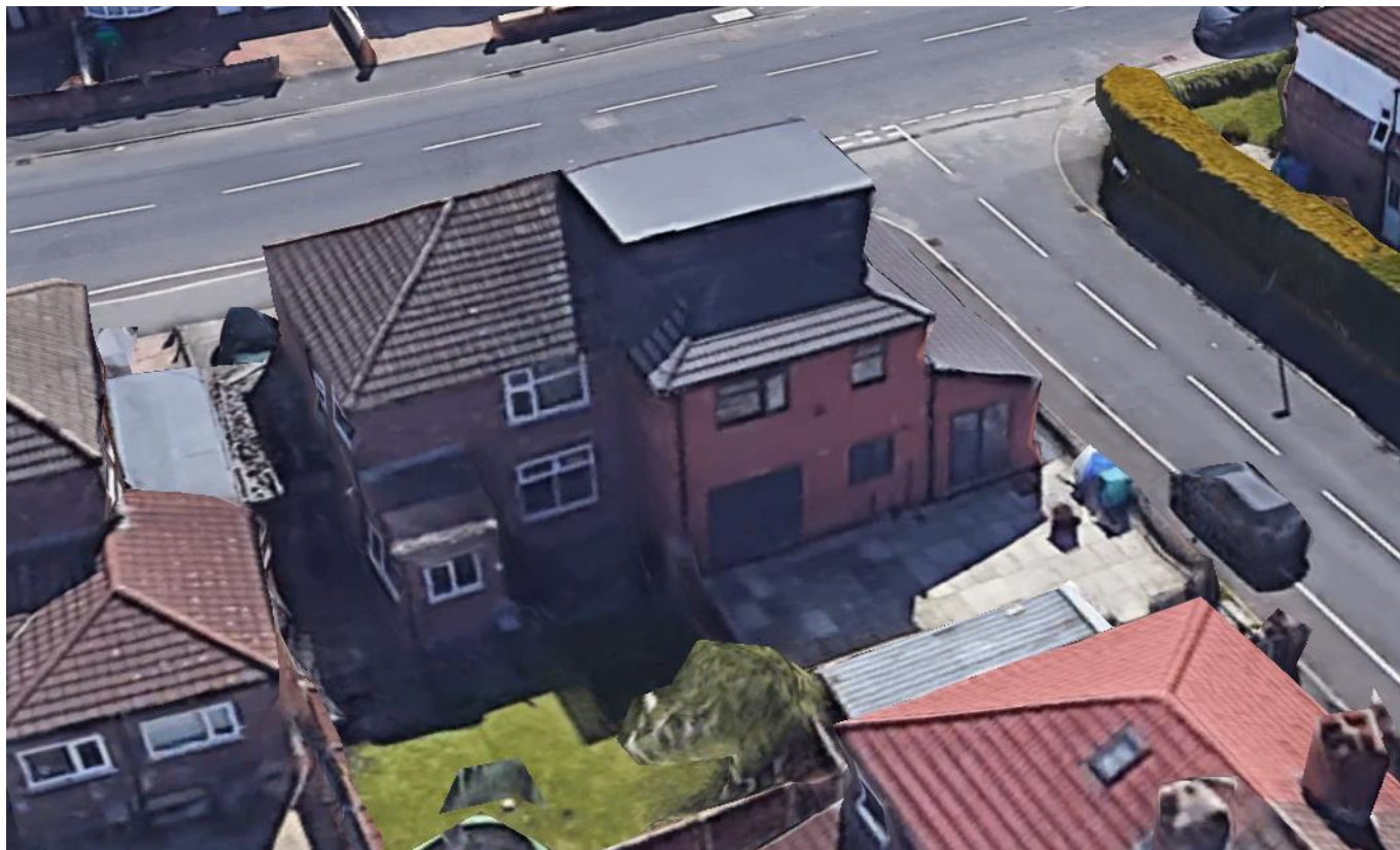
Figure 15. No.231 Mauldeth Road, as seen from Google Earth.
