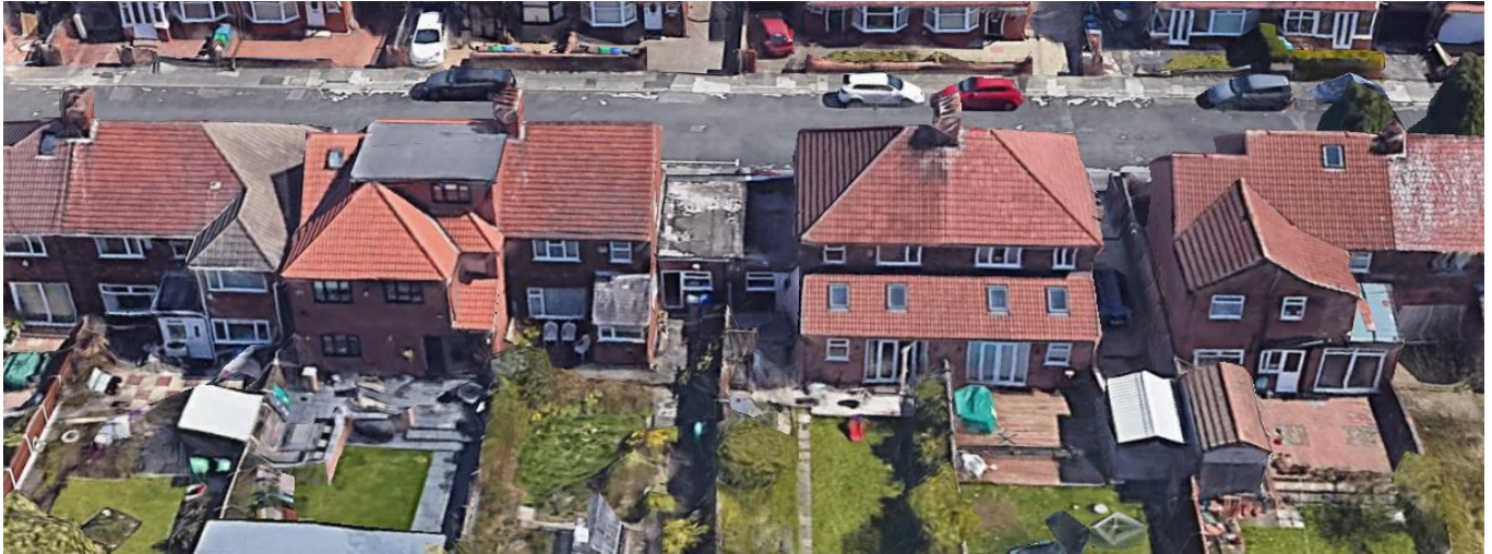
Figure 19. Properties with two-storey rear extensions along Glendale Avenue (with gaps to the shared boundary with the adjoining semi at first-floor level visible), as seen on Google Earth.
