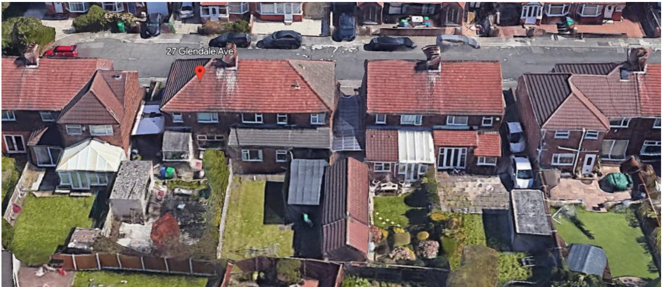
Figure 18. Properties with two-storey rear extensions along Glendale Avenue (with gaps to the shared boundary with the adjoining semi at first-floor level visible), as seen on Google Earth.
