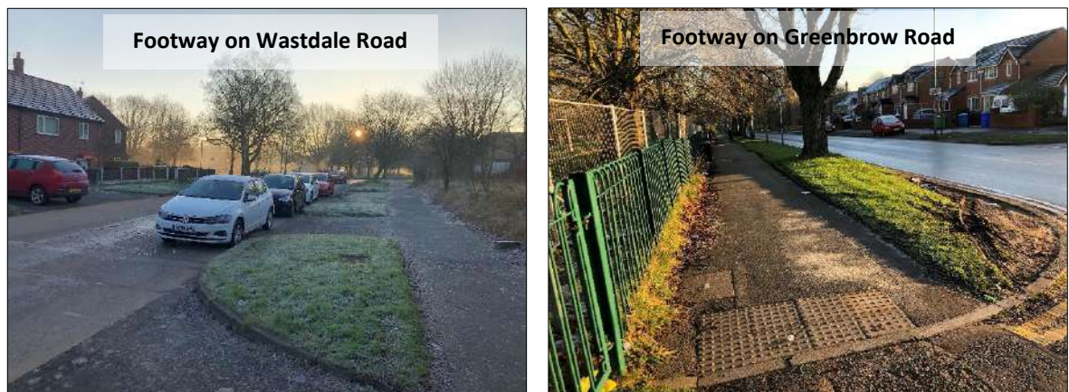
Figure 3.1: Existing Footway Provision
