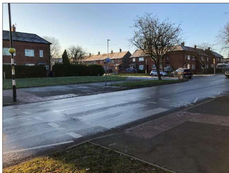
Figure 3.3: Zebra Crossing Located on Greenbrow Road
