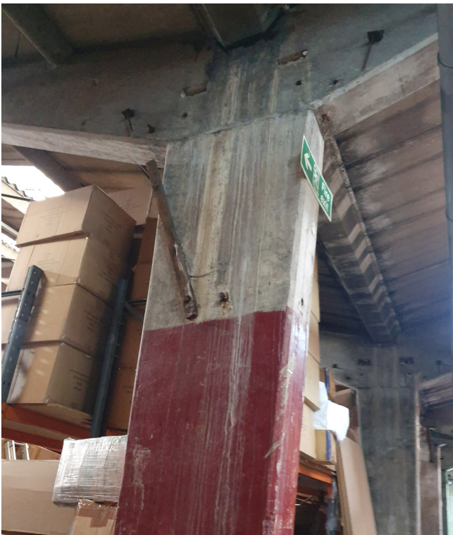
Image 03: Roof Valley Water Ingress
