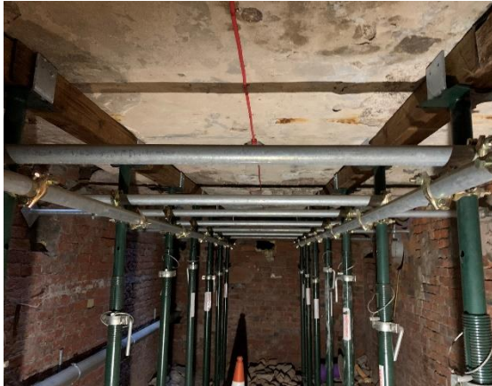
Figure 1: Temporary props supporting soffit.
