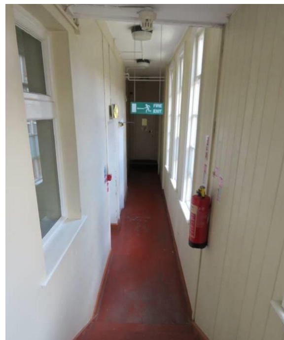
Figure 65: The interior of the narrow c1949 external corridor, which linked the rear of the council chamber to the main building.
