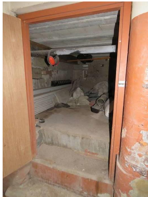
Figure 43: A small cupboard to the western end of the ginnel which was originally the location of the men's vagrant stairs. The remains of the staircase can be seen below in the basement.
