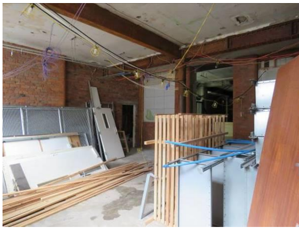
Figure 50: Looking north-west across the floor.
