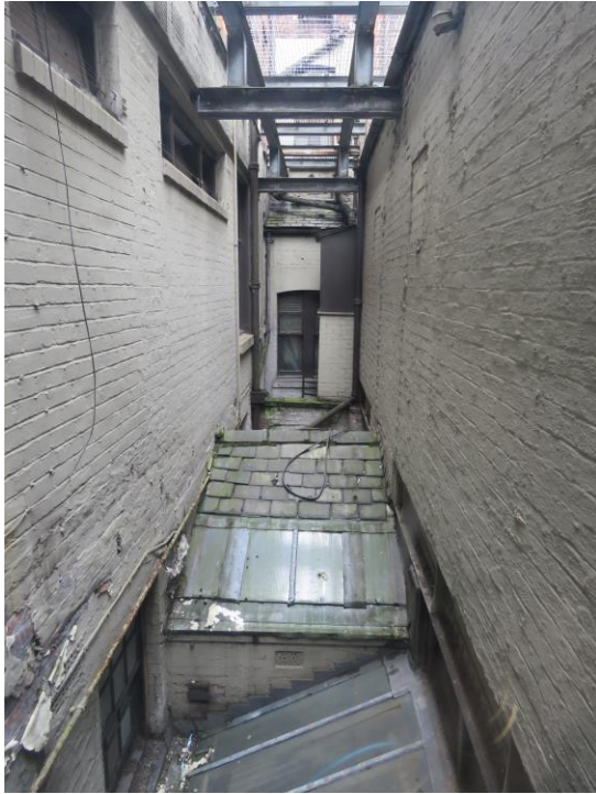
Figure 46: The central light well between the former outdoor relief waiting room (right) and remainder of the building (left).
