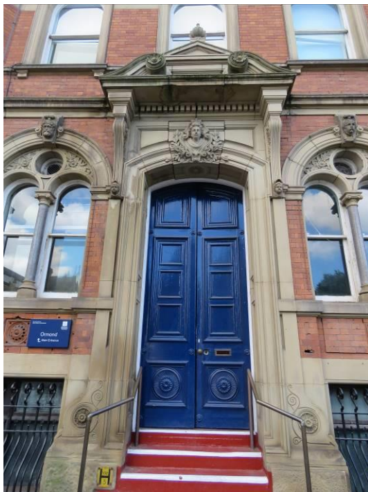
Figure 19: The principal entrance into the offices of the building.
