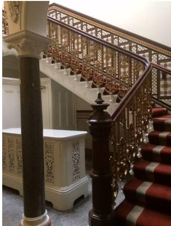
Figure 33: The principal office staircase from ground to first floors. Note the highly decorative original free-standing radiator.
