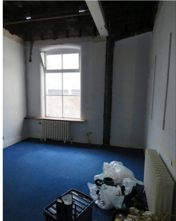
Figure 47: A room on the northern side of the outdoor relief ward which was originally part waiting room and part pay clerks glazed office and cash counter.
