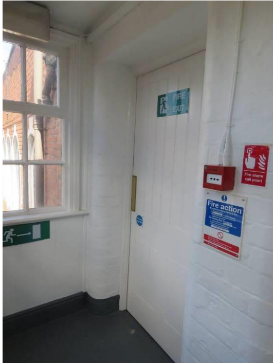
Figure 54: A typical plain battened door as found in the vagrant part of the building.
