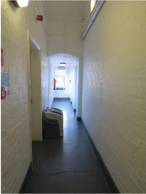
Figure 52: The first floor tramp and vagrant ward corridor, looking into the c1949 corridor extension.
