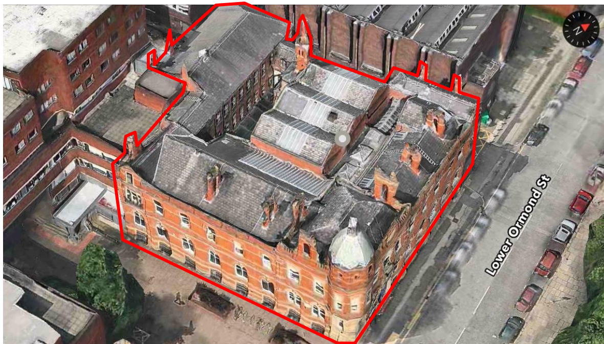
Figure 14: An aerial view looking north-west across the subject site.
