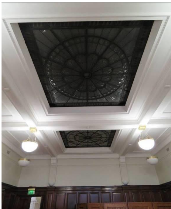
Figure 64: The c1930s ceiling lay lights which is lit by three large sky lights in the roof.
