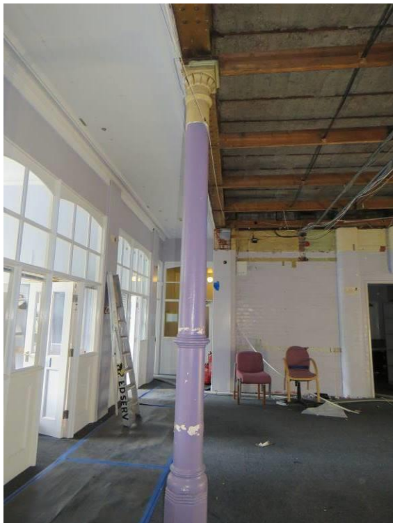
Figure 48: Looking south along the join between the original waiting room corridor (left) which is supported by a decorative cast iron column, and the altered c1920s inserted ceiling to the right, which was originally an open area.
