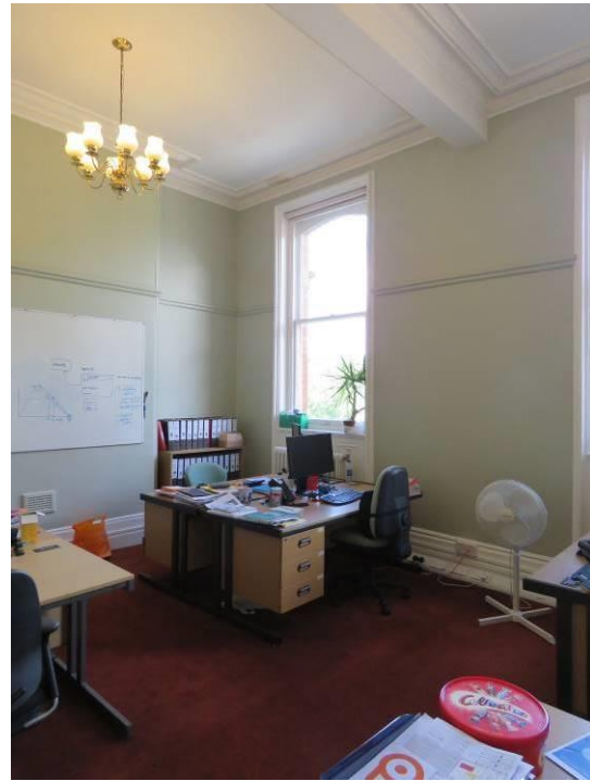
Figure 62: A typical office on the first floor, showing plain plaster cornice and picture rail.
