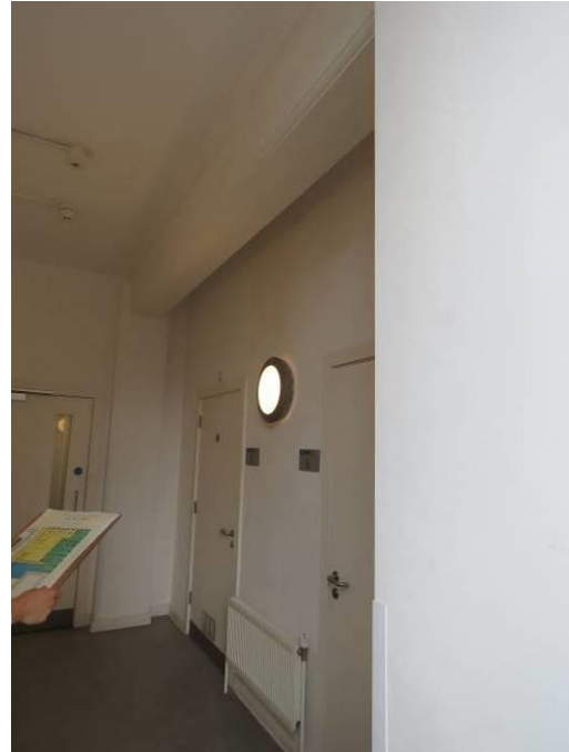
Figure 53: The altered 2006 toilets to the southern end of the formally open plan vagrant floor.
