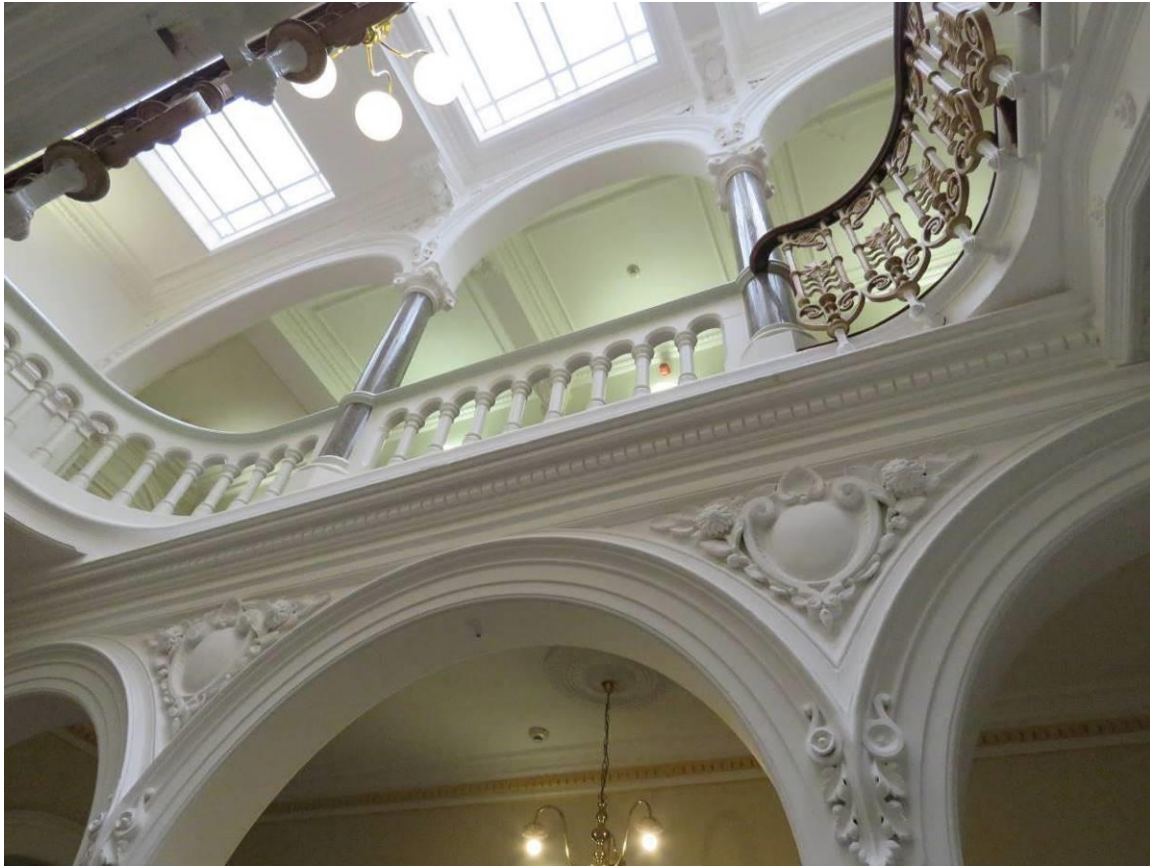
Figure 34: Looking up into the double-height staircase hall, showing the stone balustrade, carved spandrels and glazed lay lights to the ceiling.
