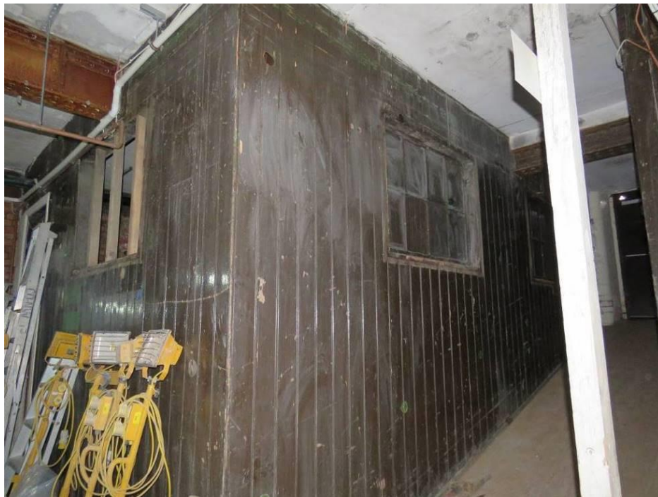
Figure 54: One of two original timber partitioned rooms, which may have been used as work rooms.
