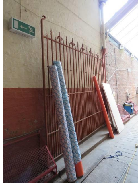
Figure 41: The secondary iron gate within the ginnel, which originally divided the vagrants from the outdoor relief.
