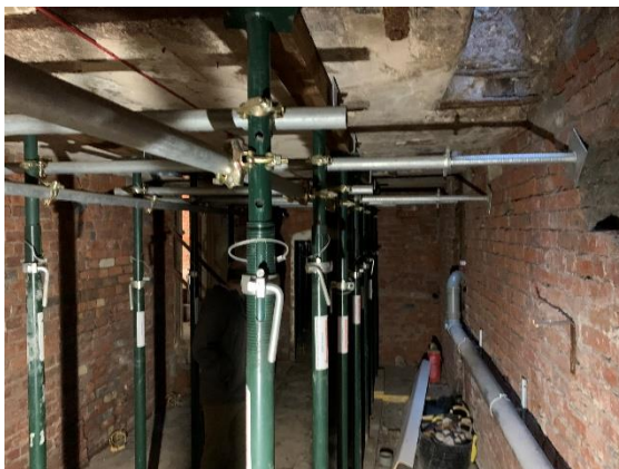
Figure 5: Temporary props supporting soffit.
