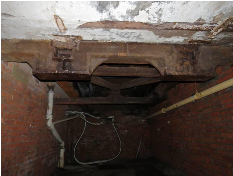
Figure 55: The underside of the original cast iron weighbridge as seen above in the ground floor cart way.
