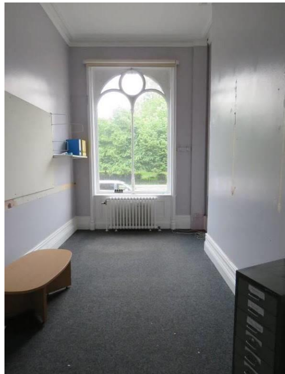
Figure 49: One of the six relieving officer's rooms to the eastern end of the outdoor relief ward. Which would have originally contained a chimneypiece to the right.
