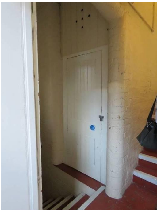
Figure 65: The simple painted brick vagrant staircase.
