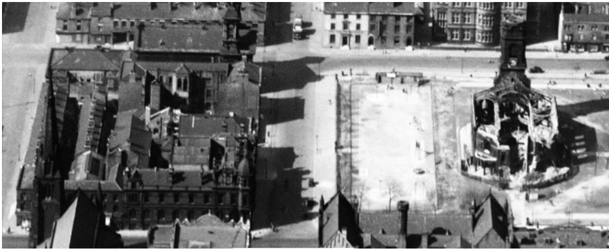
Figure 10: An aerial view looking down onto the Ormond Building from the south as seen in 1949. This photograph was taken in the year the bomb damaged All Saints Church to the right was finally demolished.
