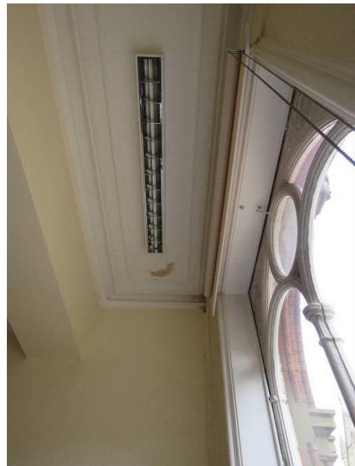
Figure 37: Looking up at the plain plaster cornice in the former corridor originally dividing an anti-room from the strong room (left).
