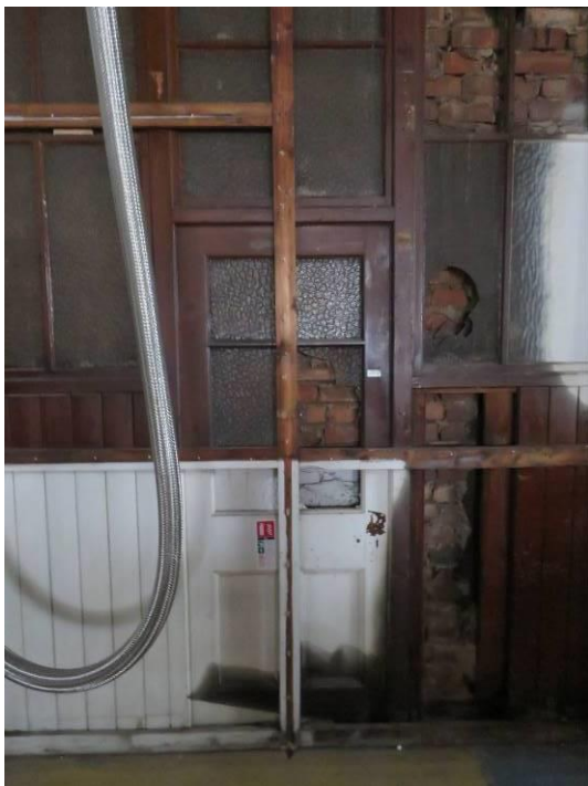
Figure 56: A previously concealed original/early glazed screen.
