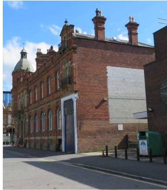
Figure 26: The north elevation from Lower Ormond Street, showing the plain nature of this façade which was originally partly concealed by the original St Augustine's Church.
