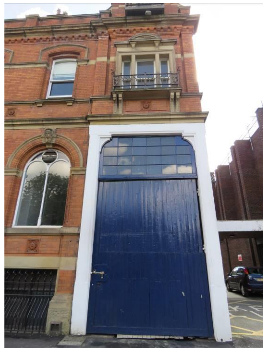
Figure 20: The cart way entrance, which retains its original cast iron gates beneath c1930s timber gate and glazed fanlight.
