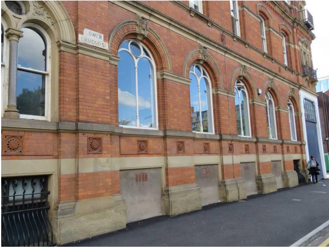
Figure 18: The lower Ormond Street elevation, which was originally used for Outdoor Relief. The cart way to the right gave sole access into this part of the building for claimants.
