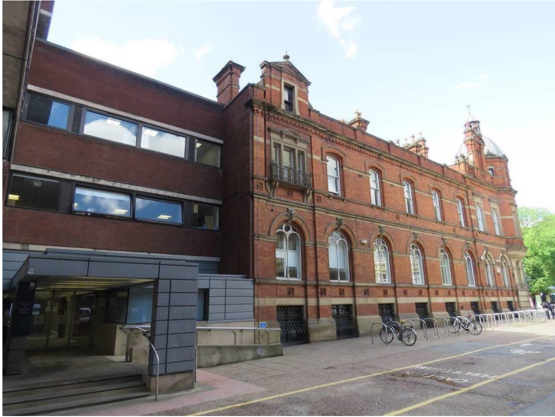
Figure 21: The Cavendish Street elevation, showing its link into the 1970s Cavendish Building to the left.
