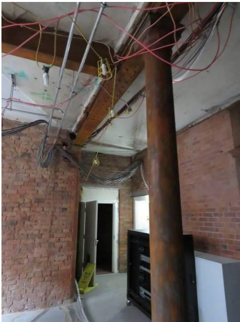
Figure 52: The sand-blasted cast iron columns and ceiling structure.
