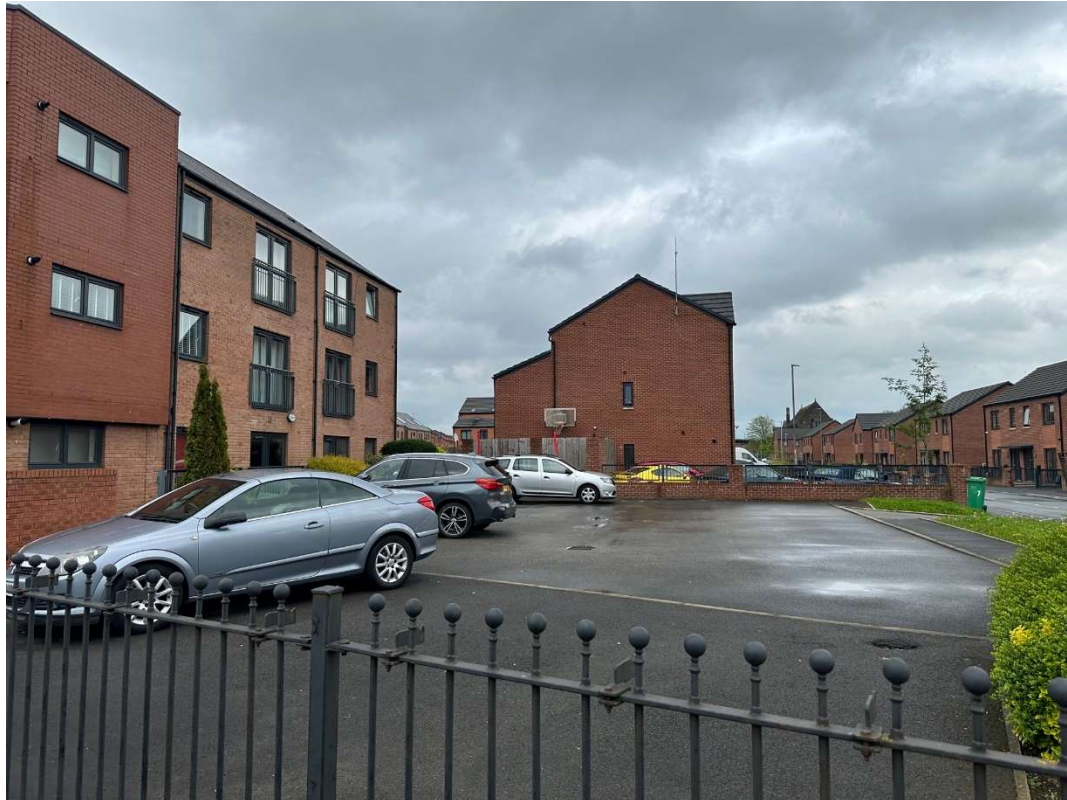
Photo of Application Site, side elevation
