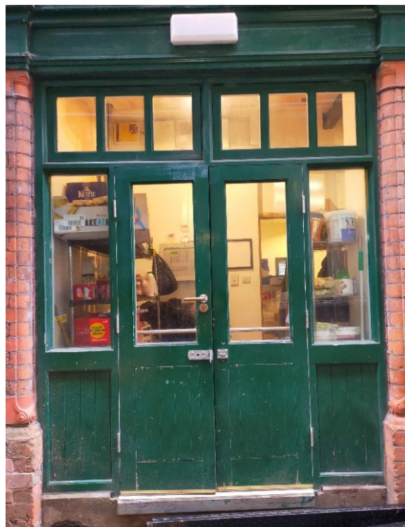
Existing fire exit door - Exterior
