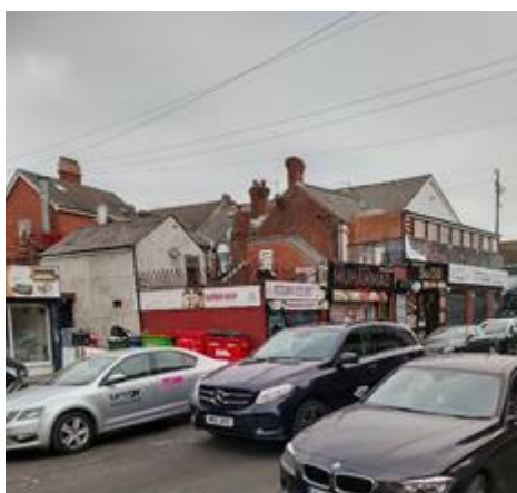
Fig.1 – Views of the application site with existing railings in situ.
