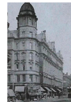
A photograph of the site in 1905, showing original fabric awnings inserted within the window openings to the ground floor
