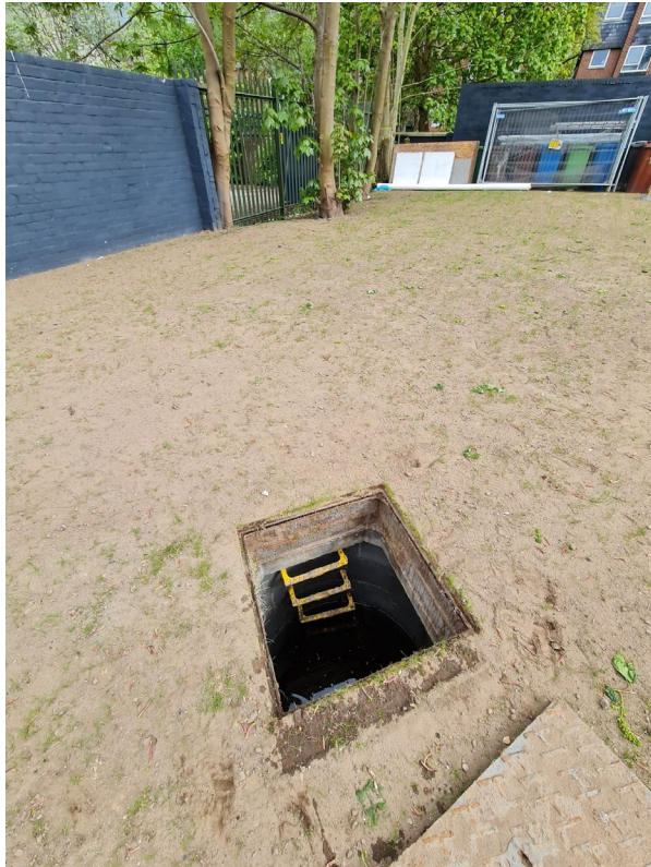
Suds4 Completed works – Silt Trap Photo taken 5th May 2023
