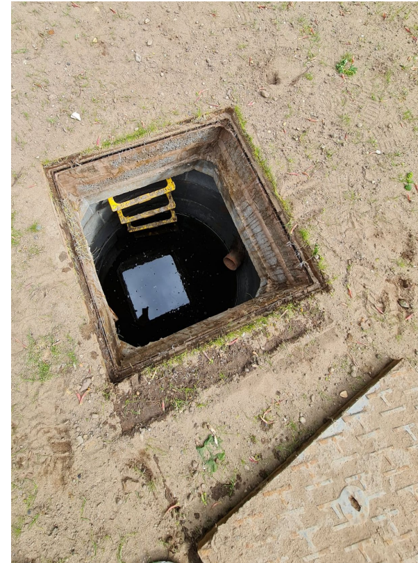
Suds5 Completed works – Silt Trap Photo taken 5th May 2023
