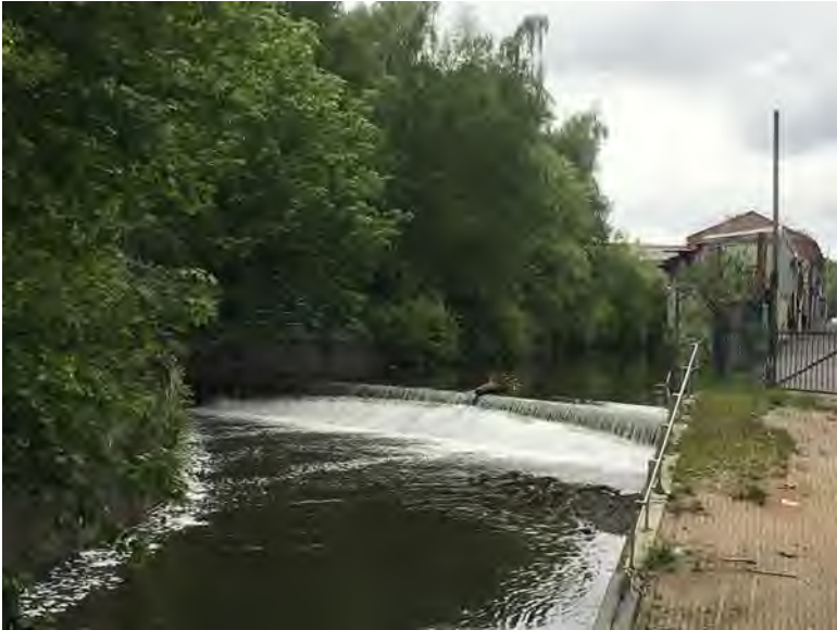
Photo 1: Looking upstream along the River Irk, approximately 0.4km upstream of the application boundary. Photo shows reinforced riverbank, overgrowth vegetation on the right bank of the river and a weir stretching across the channel.
