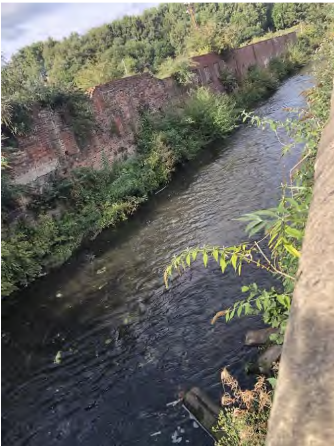
Photo 4: Photo looking upstream along the River Irk, approximately 500m from the application boundary. Photo shows protruding vegetation through riverbank walls.
