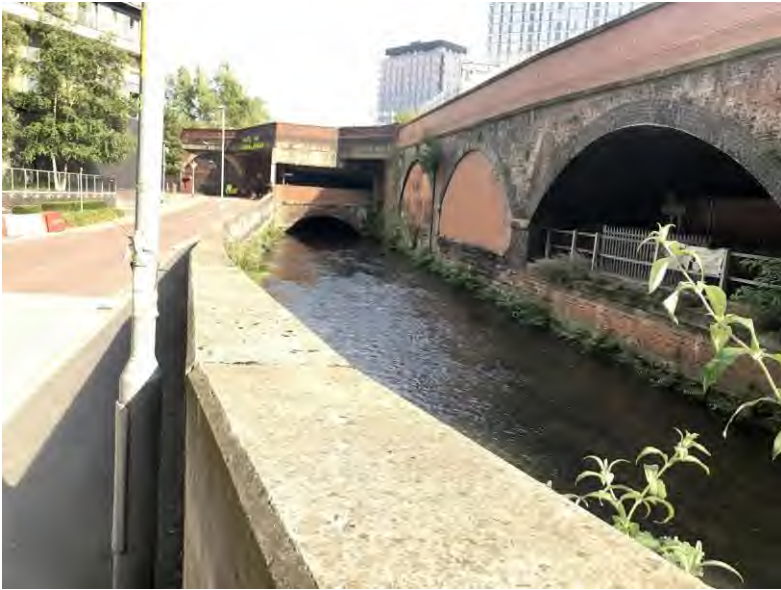
Photo 3: Photo taken on Dantzig Street looking upstream along the River Irk, on the right riverbank. Photo shows highly modified riverbank with a brick wall either side. Photo shows outlet of concrete arch culvert, dimensions unknown.
