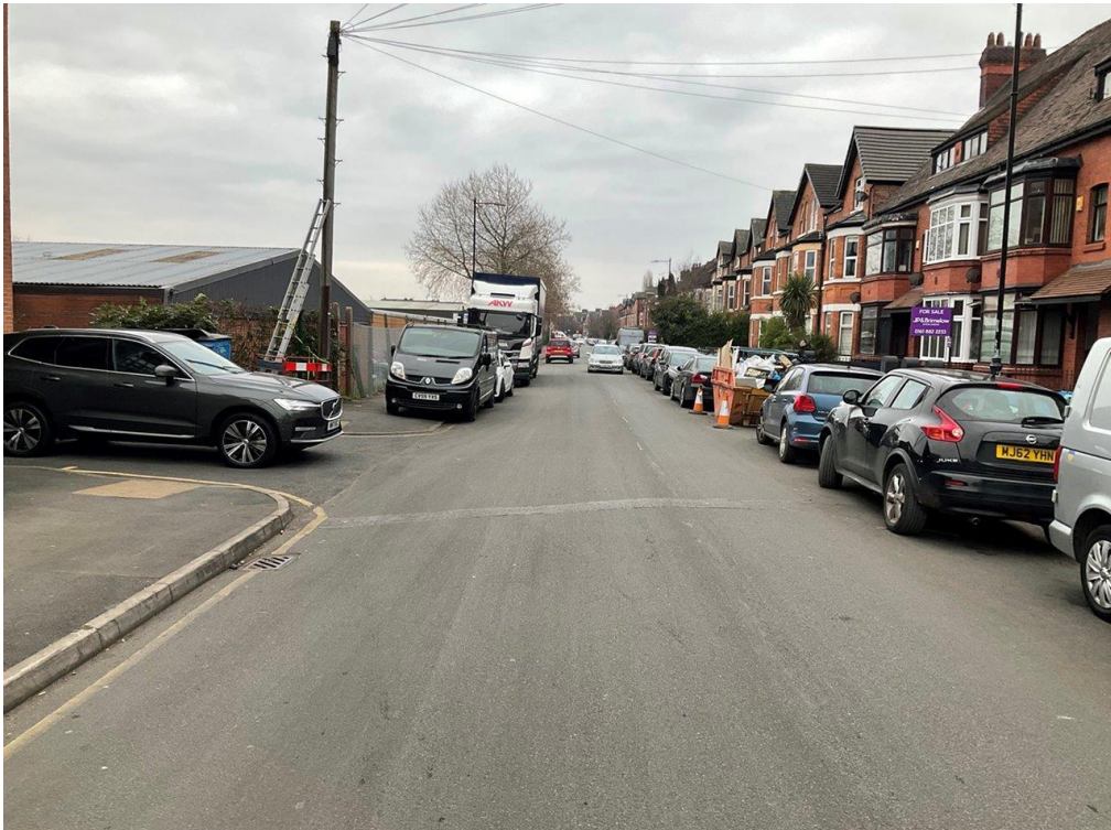
6.2 General view looking south on Albany Road
