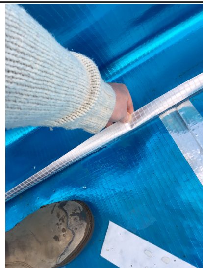
Double sided butyl tape sealing lap
