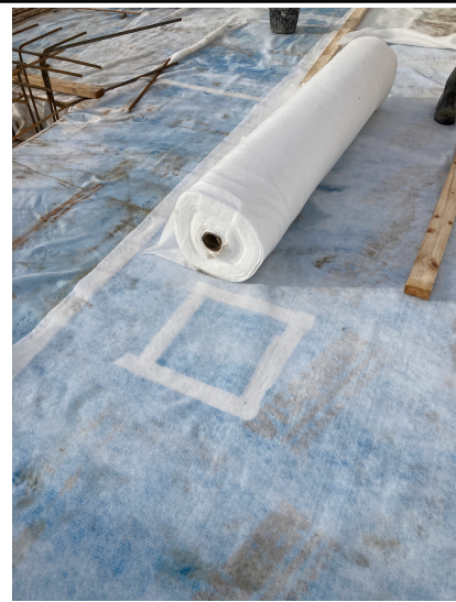
Protective fleece applied to membrane
