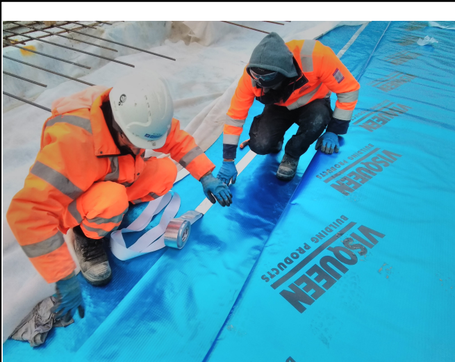
Installers applying double sided butyl tape
