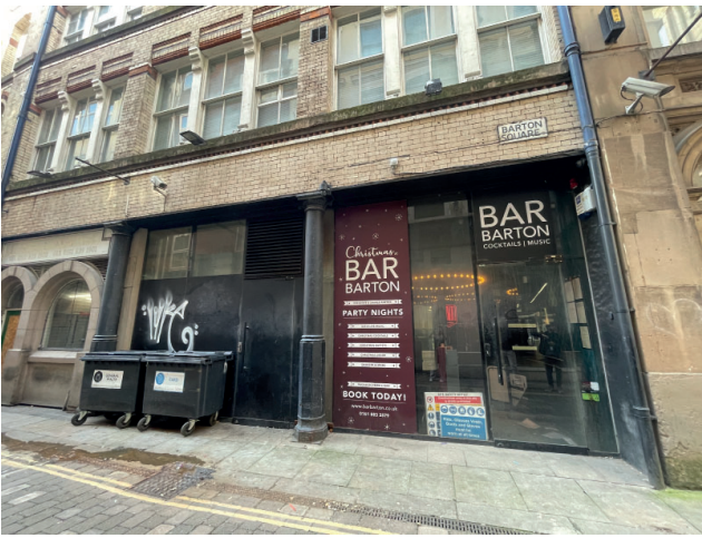
EXISTING EXTERNAL PHOTOGRAPHS
