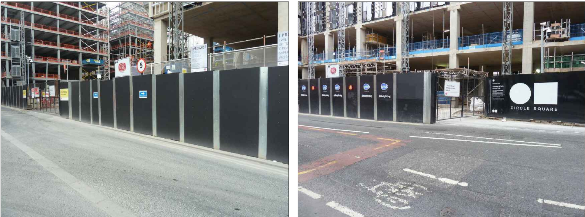
EXAMPLE OF HOARDING TO BE USED ON SITE
