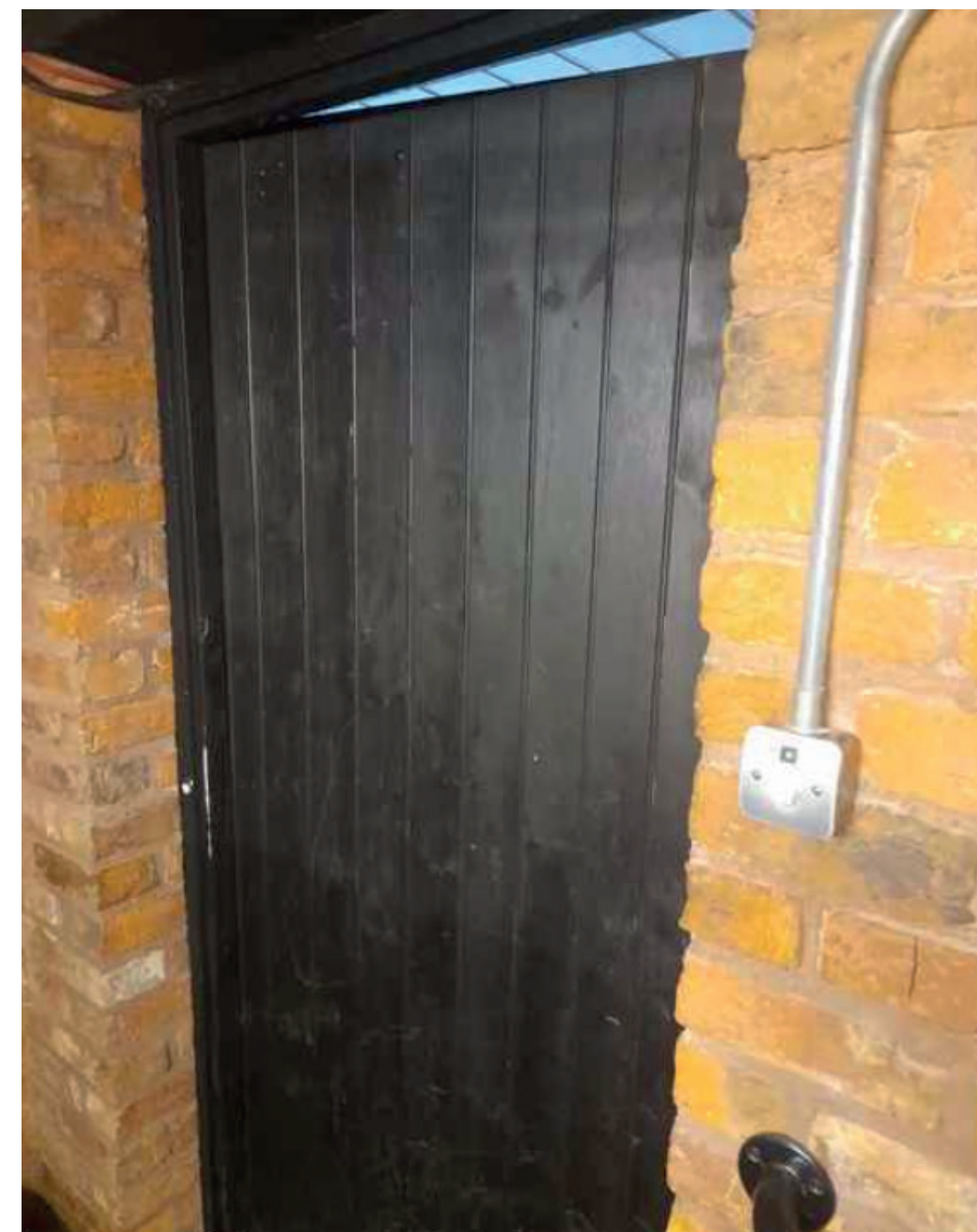
Typical existing vertical boarded timber door
