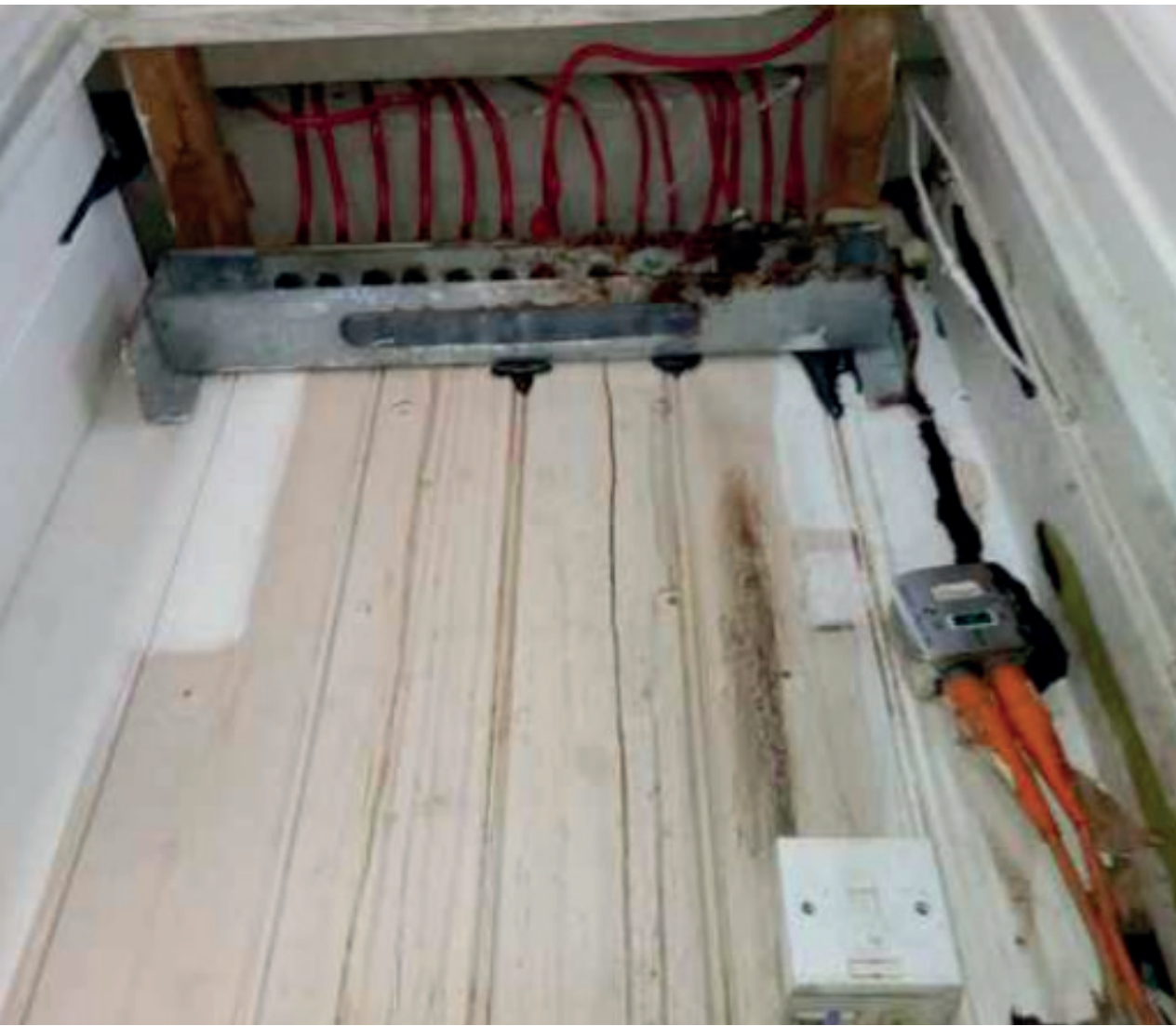
Example photo of existing wall recessed cupboard to be lined
