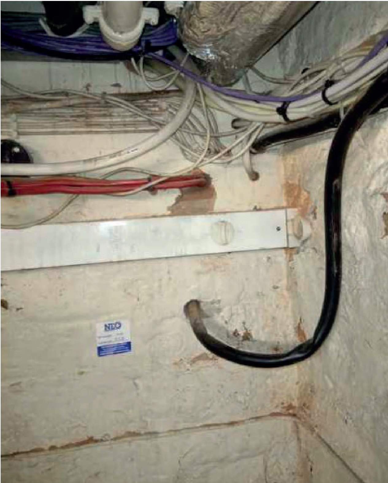
Location of localised cleaning of brickwork to enable standard fire stopping detail to be installed.
