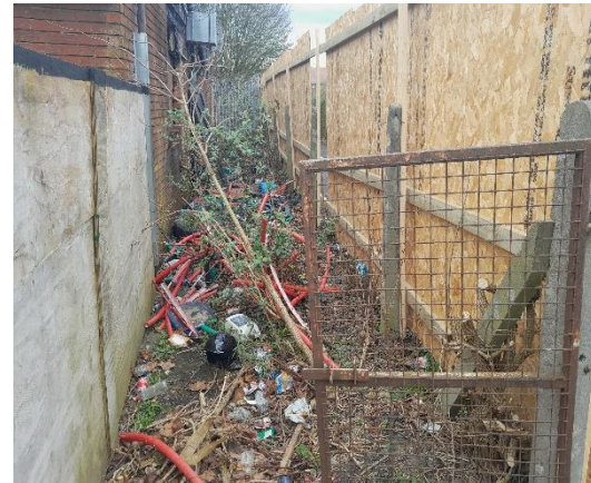
Photo 10: Strip adjacent building and boundary.jpg
