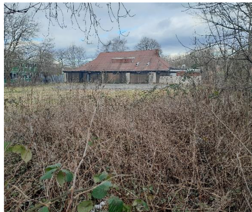
Photo 4: Site overview to club building
