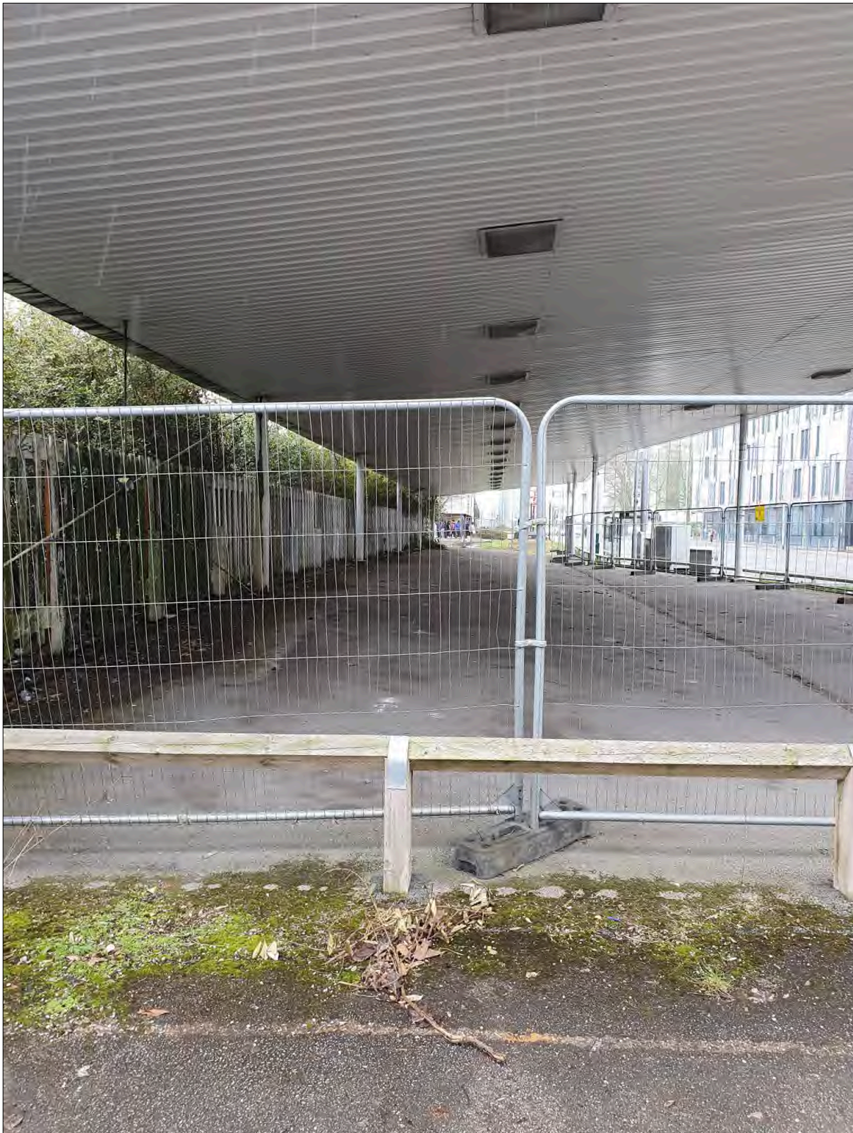
Plate 15 Photograph of disused car sales structure, facing south-east
