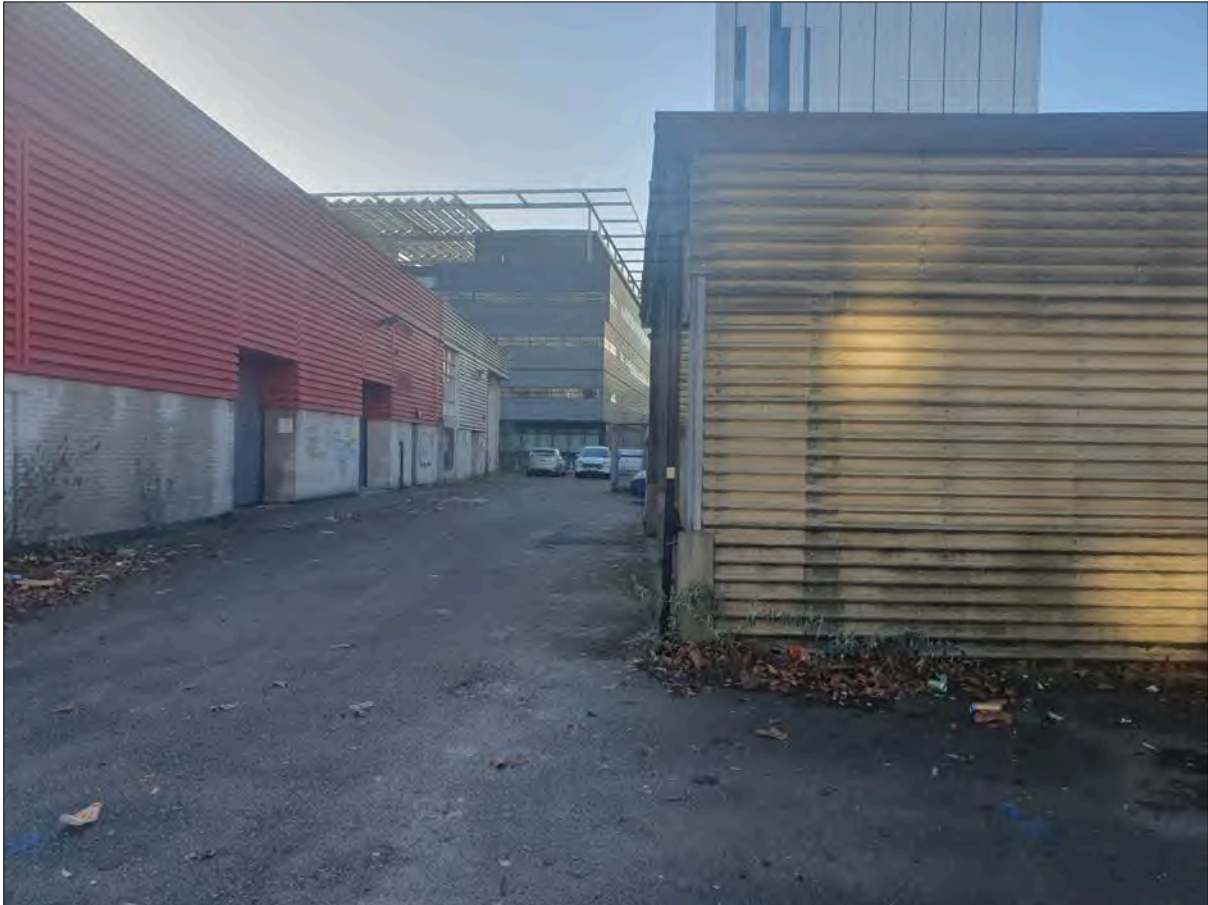
Plate 13 Photograph showing the plastic cladded shelter in the north of the Site, facing south.
