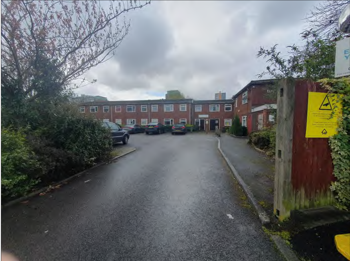
Plate 16 Photograph of Elizabeth Yarwood Court, facing south-west
