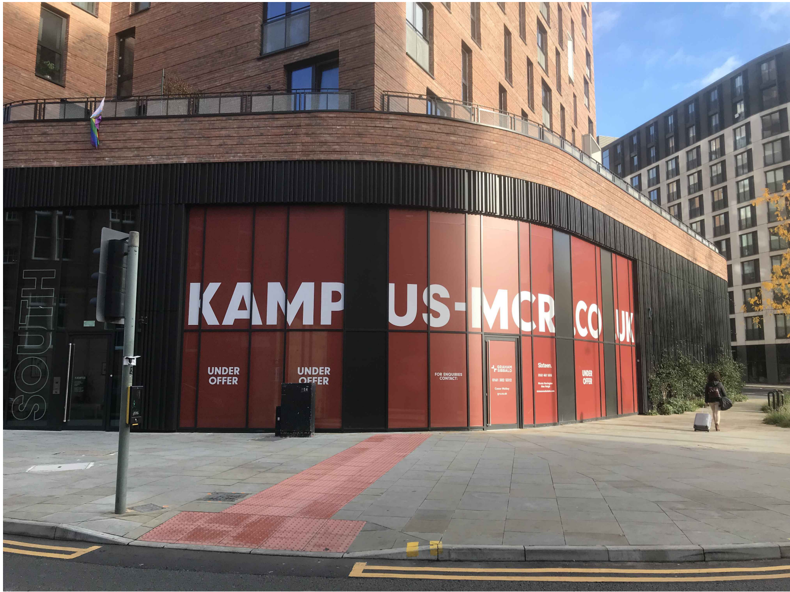
03 EXISTING PHOTOGRAPH 030 NTS
