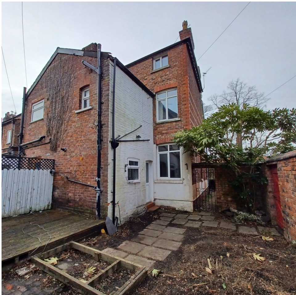
Figure 2. Rear view of No.34 Cavendish Road.
