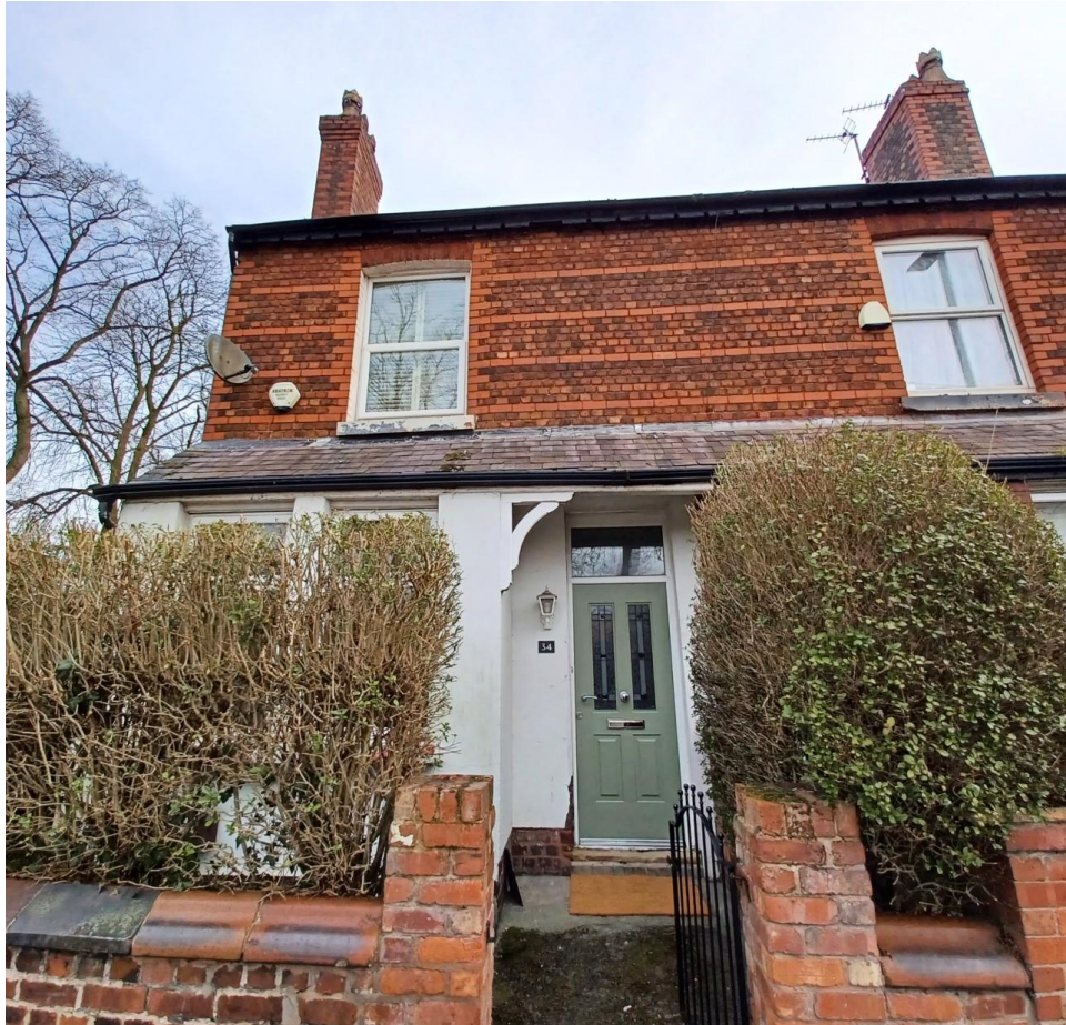
Figure 1. Principal elevation of No.34 Cavendish Road.
