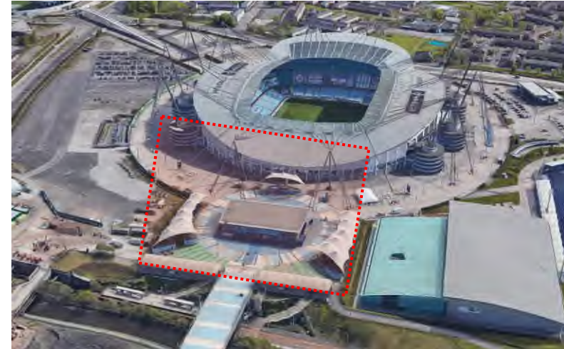
Figure 01: Existing Etihad Stadium with project area highlighted (Source: Google Earth)
