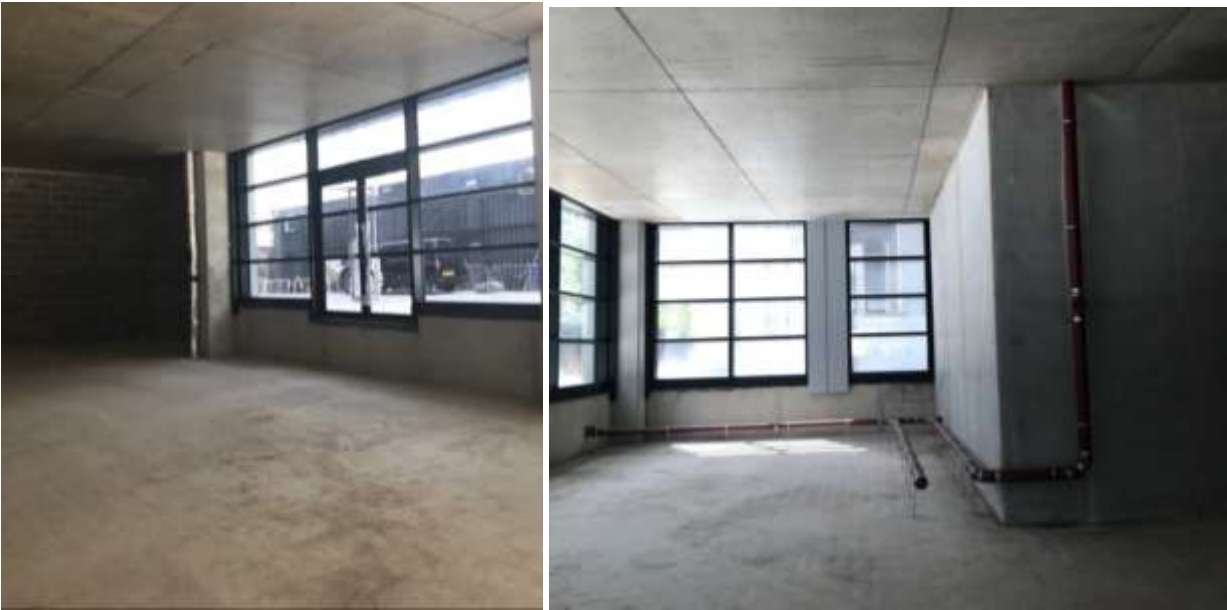
Figure 3 Photographs of ground floor base build unit
