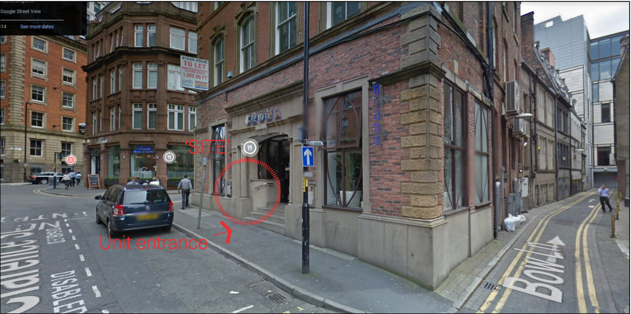
Fig. 01: Site location, showing existing steps to entrance to unit. The proposal is for an external wheelchair lift to a section of non original fabric
