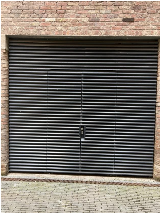
Current bin store door at Crusader which is the same proposed at Neptune.
